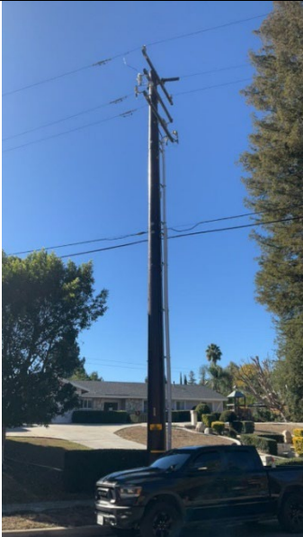
Item10GIimg1: Overall pole.
