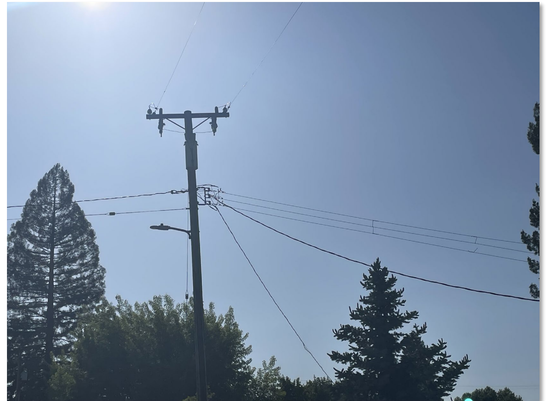
Secondary splitting into multiple services
