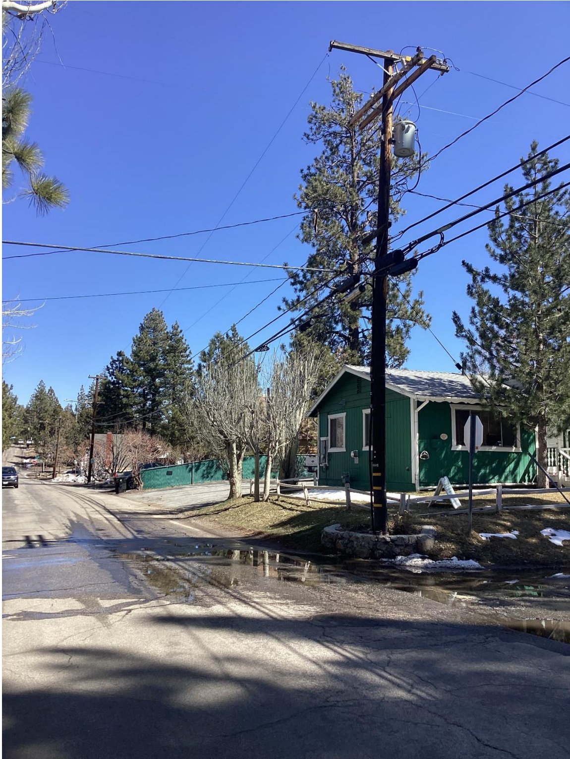
After Trimming on January 25, 2024
