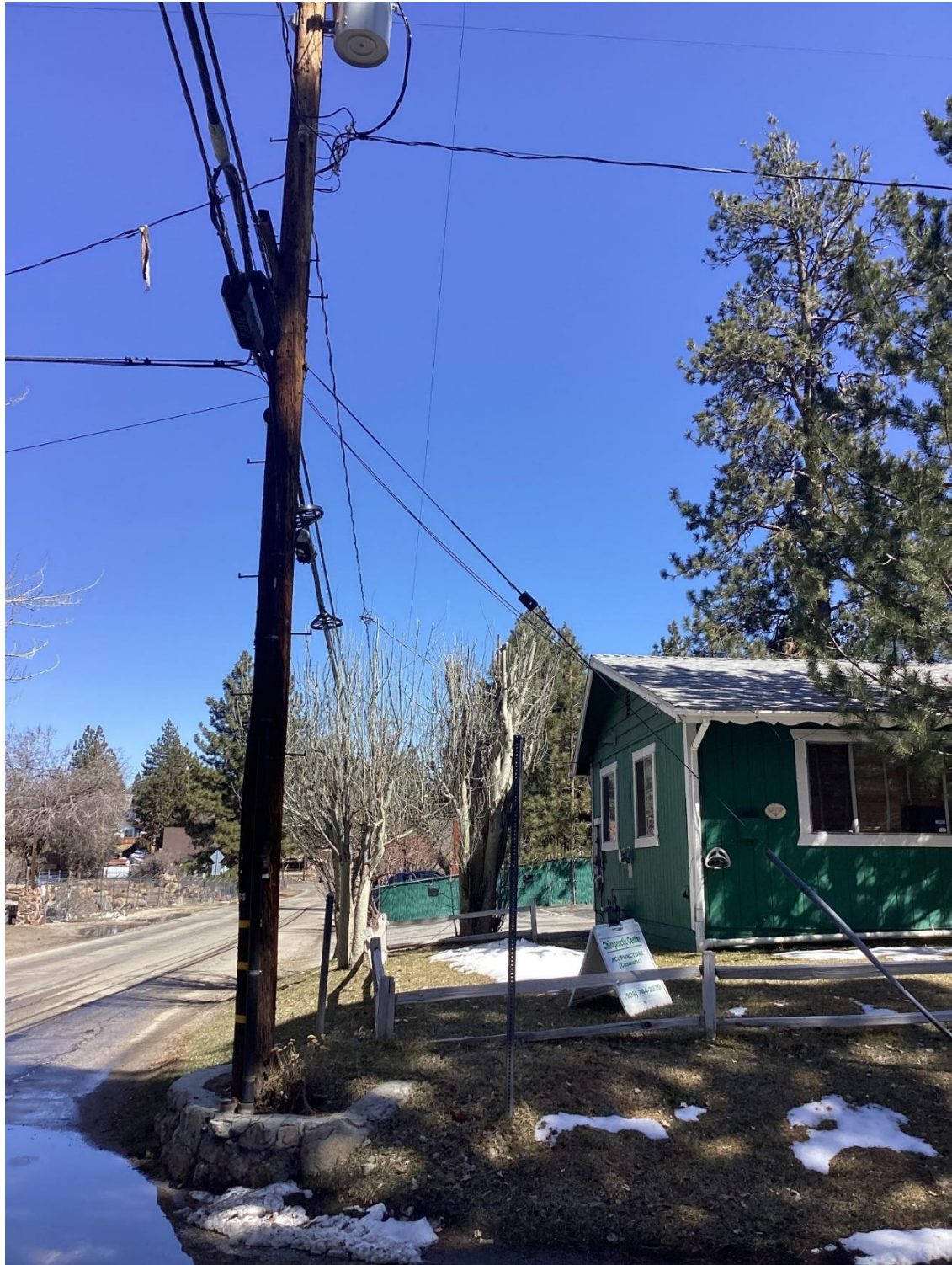
After Trimming on January 25, 2024
