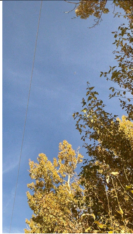
Item2IA1Img2: View of cottonwood limbs approximately four to five ft from a primary conductor.
