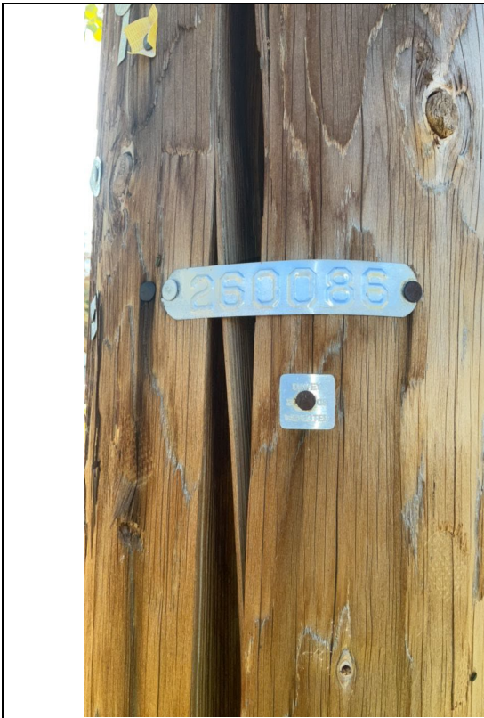
Item4Gimg1: Pole ID.
