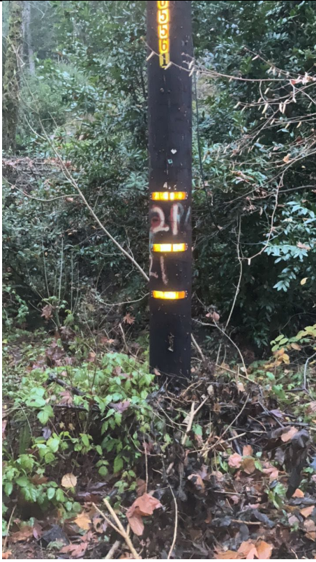
Item14IA1img2: Live vegetation within the firebreak 10-foot radial clearance.
