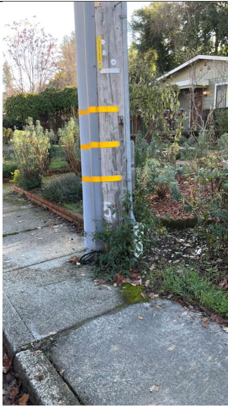
Item6IA1Img1: Live vegetation within 10-foot radial clearance.
