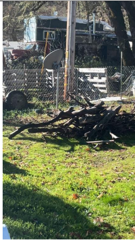
Item1IA1Img1: Other view of wood pallets within the 10 ft firebreak radius of pole.
