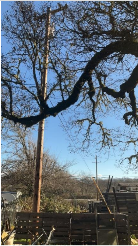
Item1GImg3: View of wood pallets in foreground within 10 ft firebreak radius of pole.
