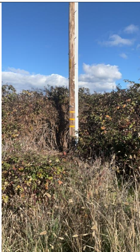
Item3IA1Img3: Large angle view of heavy blackberry growth within the 10 ft firebreak radius of pole.
