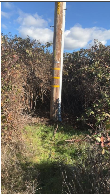
Item3IA1Img2: Heavy blackberry growth within the 10 ft firebreak radius of pole.
