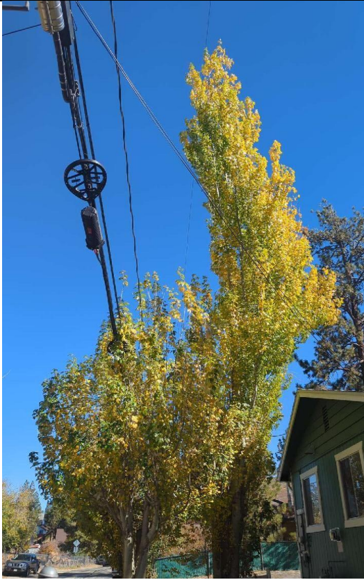
Item15IA1img1: View of tree growing within the 72-inch safe clearance distance of the conductor.
