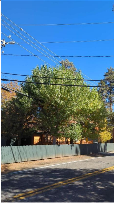
Item10IA1img1: Overall view of tulip tree in contact with covered conductor.
