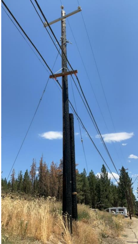
Item1GImg1: Overall Structure
