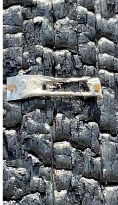
Item1GImg2: Structure ID 294723
