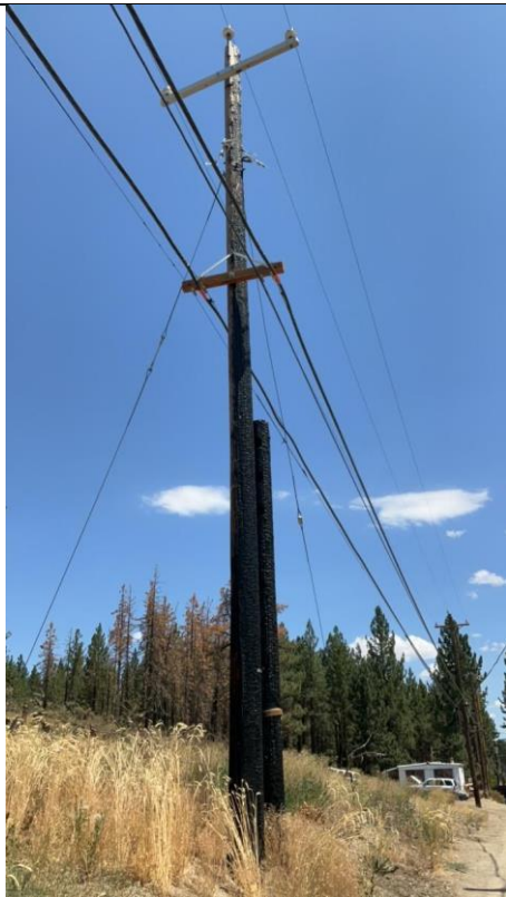
Item1GImg1: Overall Structure
