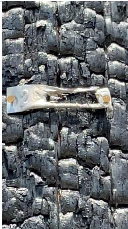
Item1GImg2: Structure ID 294723
