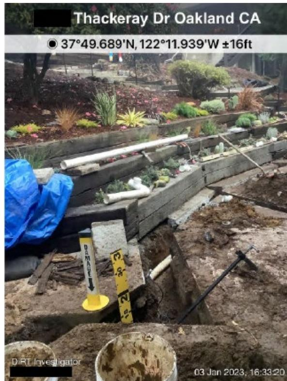
Photo 4: Photo from the PG&E Investigation Report depicting the location and a measurement of the depth of the damaged facility. Redaction by PG&E. (Exh. 4.)
