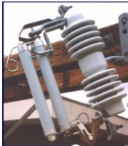
Figure SCE 8-07 - Example of Current Limiting Fuse and Fuse Holder
