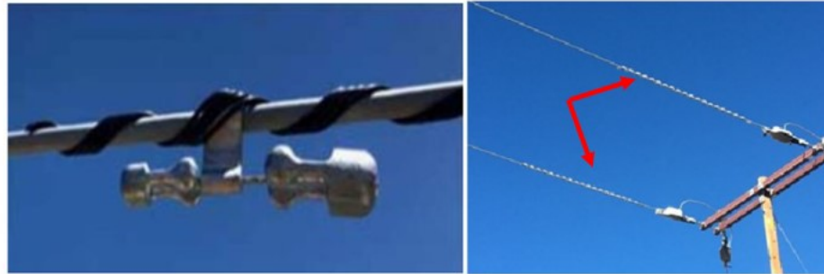
Figure SCE 8-03 - Types of Vibration Dampers: Stockbridge Damper (left) and Spiral Damper (right)
