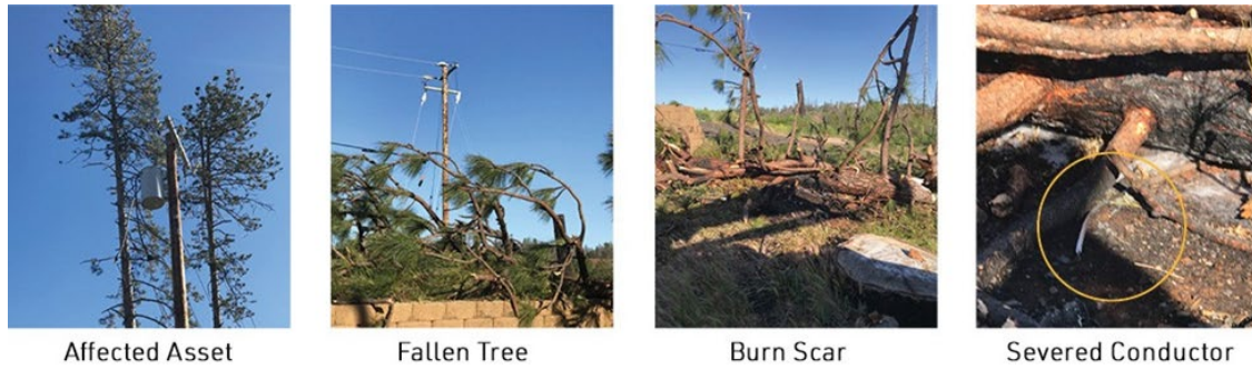
Figure F-2 PG&E Covered Conductor Effectiveness – Example 1
