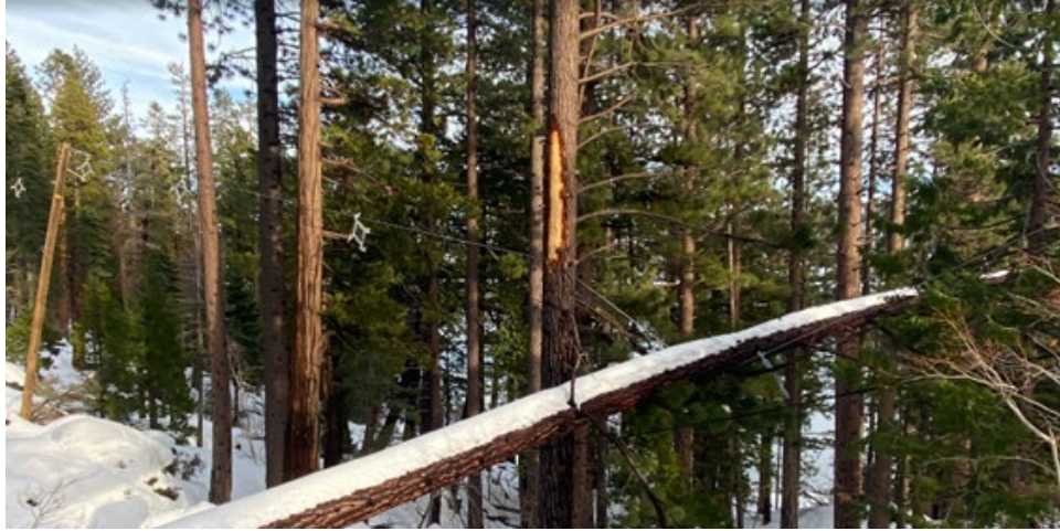
Figure F-6 Liberty Spacer Cable System Preventing a Fault – Viewpoint 1
