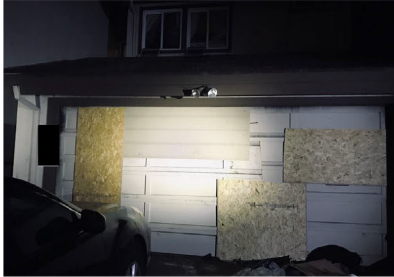
Photograph 2: Taken by the troubleman on June 21, 2020 of the outside of the Incident Location and boarded garage
