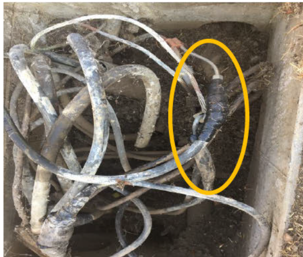
Photo 5: Taken on October 4, 2021 of the neutral splice repair previously made by the troubleman
