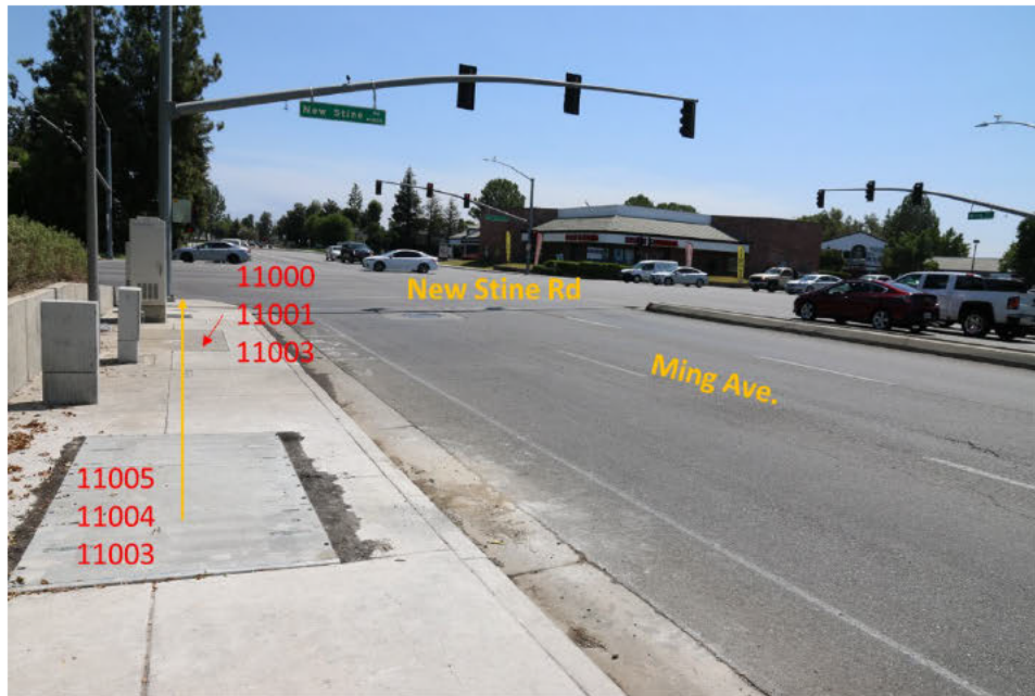
Figure 10: Location of the 3-way switches – the switch failed catastrophically on July 25, 2020. Photo taken on August 4, 2020.
