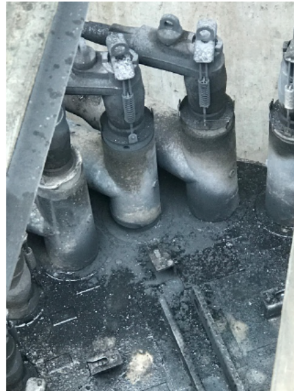
Burn mark on SW-14931 and the connectors - close-up view
