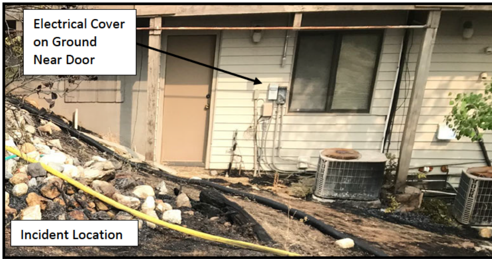
Figure 6: 09/09/22 PG&E troubleshooter image obtained post-incident of AC units at Incident Location
