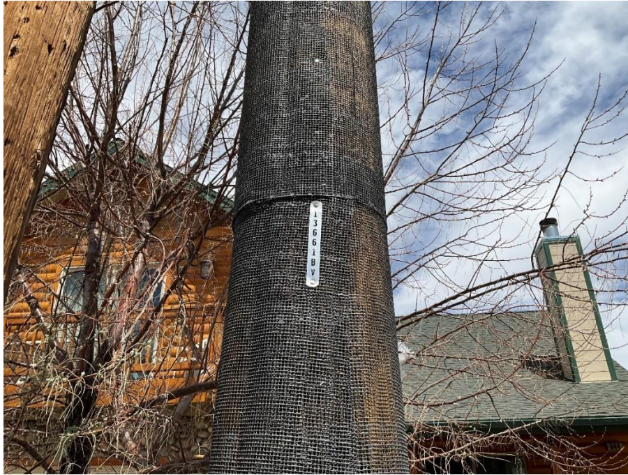
Figure 2-13 — Representative Photo of a Pole Fire Wrap Installation
