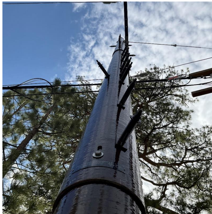
Figure 2-19 — Representative Photo of a Pole Replacement (Wood to Composite)
