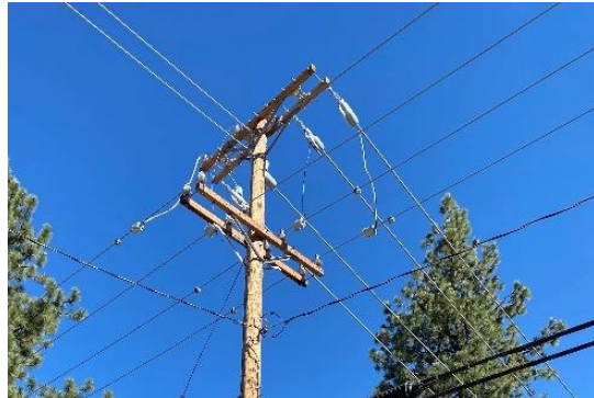
Figure 2-22 — BVES Wooden Pole #14028BV and installed Fault Indicators
