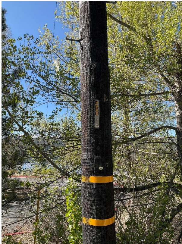
Figure 2-13 — Representative Photo of a Pole Fire Wrap Installation
