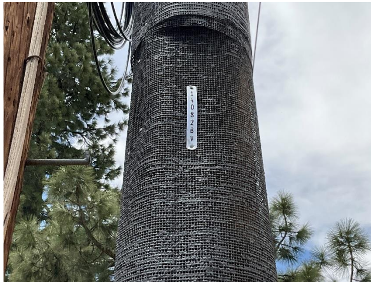
Figure 2-11 — Representative Photo of a Pole Fire Wrap Installation
