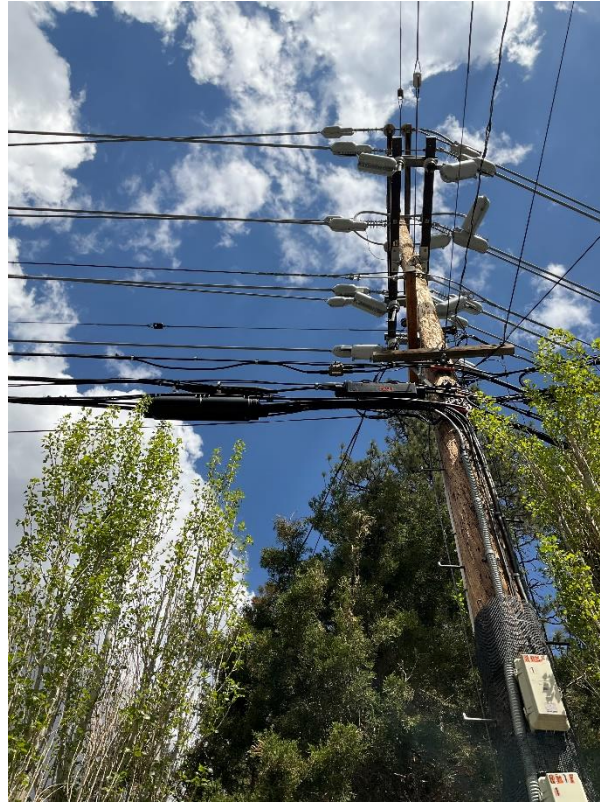
Figure 2-11 — Representative Photo of a Pole Fire Wrap Installation
