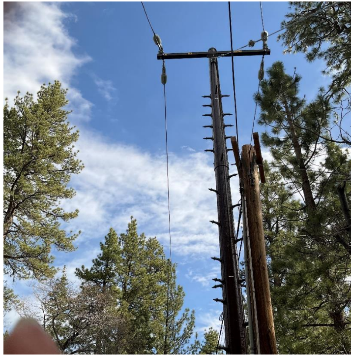
Figure 2-19 — Representative Photo of a Pole Replacement (Wood to Composite)
