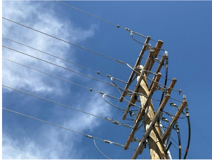
Figure 2-8 — Representative Photo of Fault Indicators Installed on Pole
