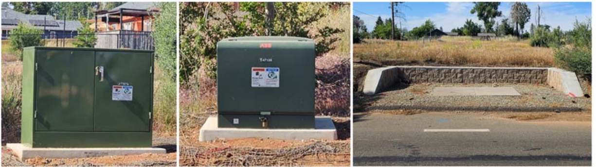
Figure 10: Example Undergrounding Assets Field Image
