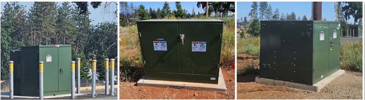
Figure 12: Example Undergrounding Assets Field Image
