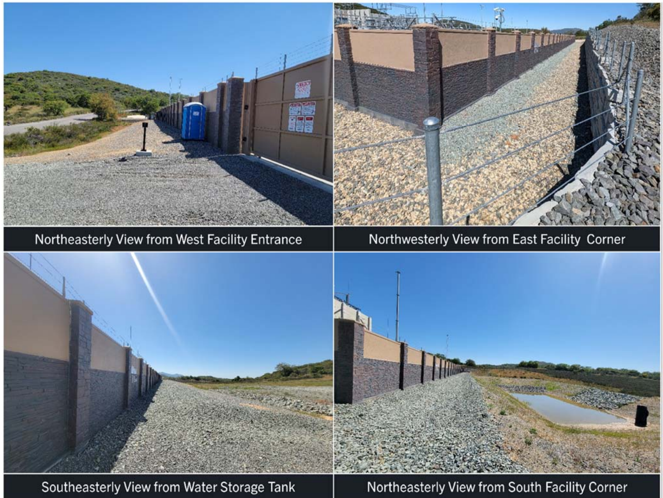
Figure 4: HWT [REDACTED] Perimeter 30-ft Fire Rock Break
