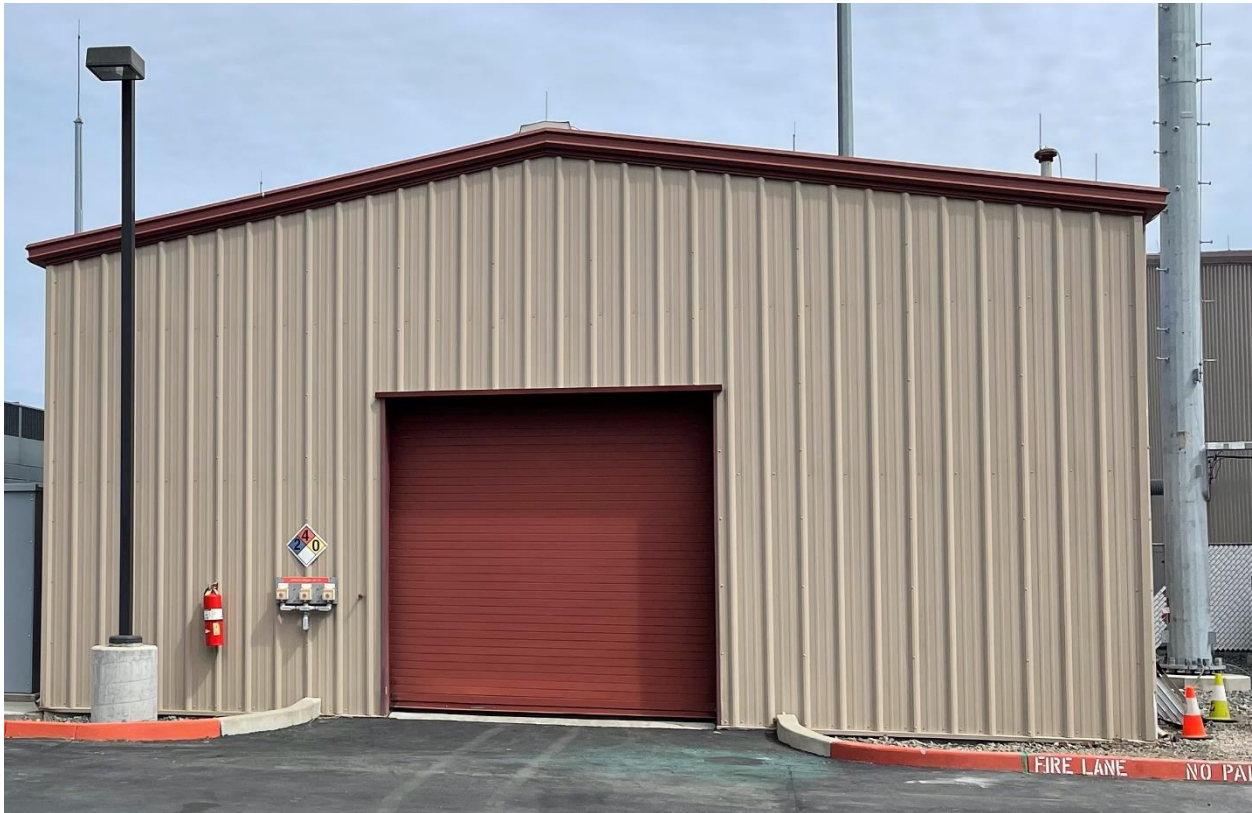
Figure 12: Spare Parts Building
