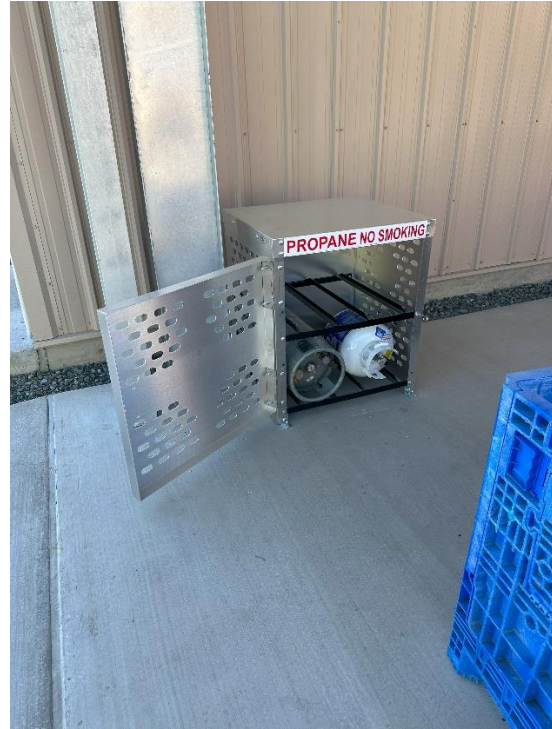
Figure 9: Compressed Gas Storage Cage
