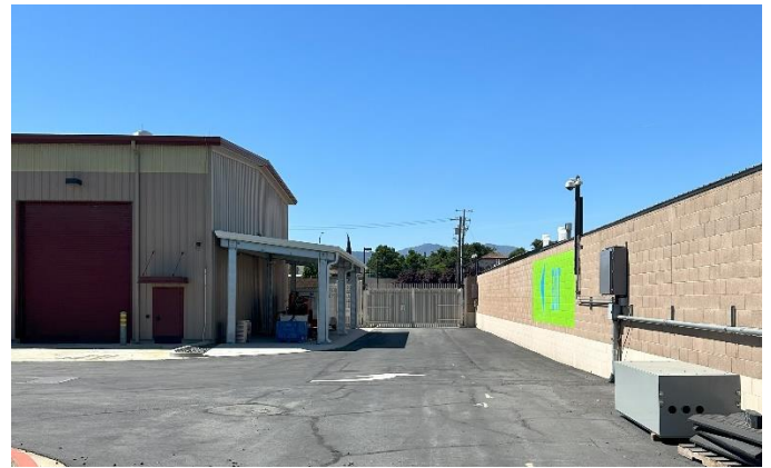
Appendix Figure 2: Receiving Warehouse Foam Trailer Storage and SW Exit Gate
