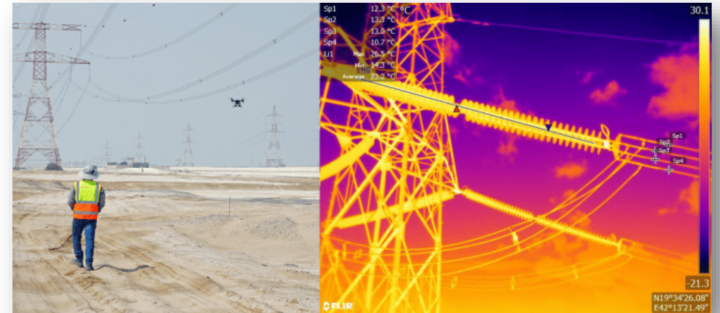
Image source: Drone Power Solutions. "Drone Inspections Are Improving Efficiency in the Utilities Industry." Leading Drone Company | Drone Service Provider, 23 Sept. 2020, feds.ae/drone-inspections-in-utilities-industry/
