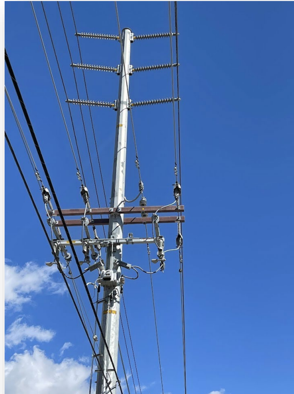
Image source: Green Grid Inc – Underbuild distribution pole
