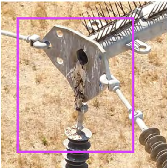
Figure 71 Damaged raptor guard (left). Poles with open-ended crossarms with evidence of bird activity should be covered as in the photo (right). If not, they should be written up with an F priority tag.
