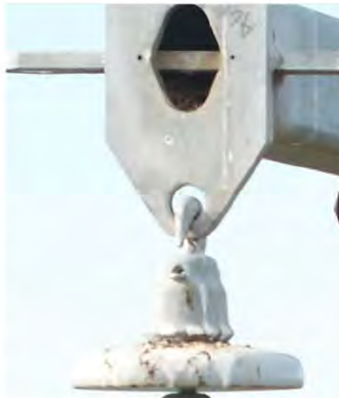
Figure 71 Damaged raptor guard (left). Poles with open-ended crossarms with evidence of bird activity should be covered as in the photo (right). If not, they should be written up with an F priority tag.
