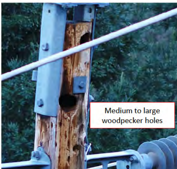
Pole cracks/rot with material loss (left). Single pole deflection on H-frame (right).
