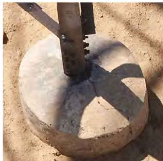
Figure 228 Rebar exposed with > 50% material loss (left). Foundation crack exceeding 1/2" in width AND extended to the stub (right).
