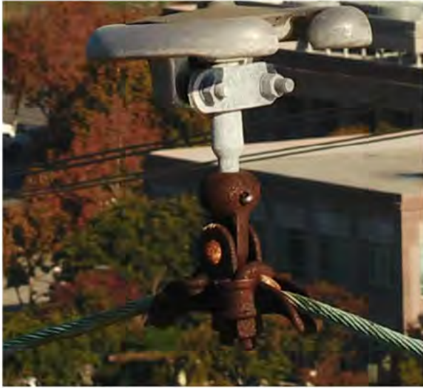
Condition: 1 Priority: No notification required
