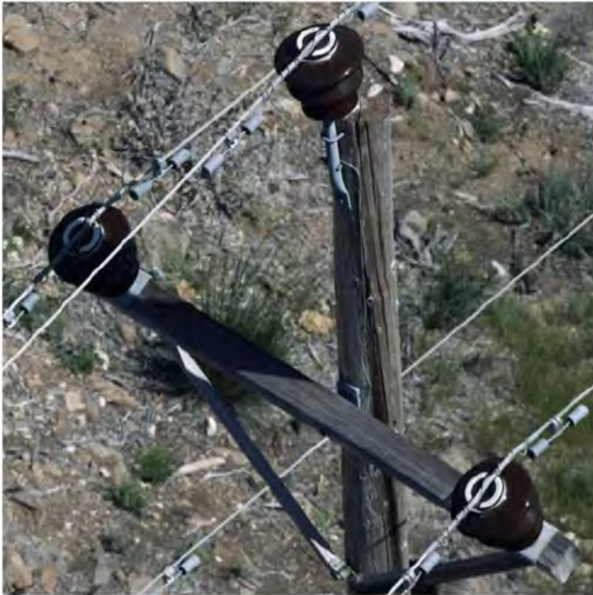
Figure 67 Crossarm cracked >50% (left). Crossarm cracked/rotten with signs of hardware slippage (right).
