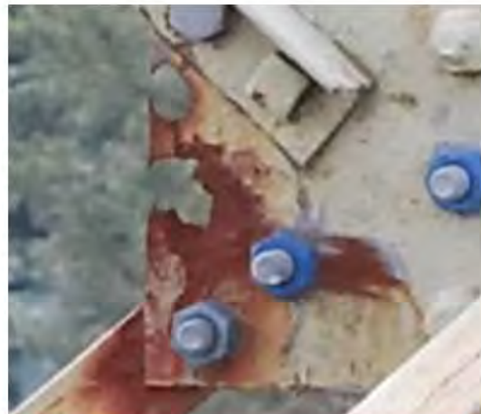
Figure 77 Severe member rust (left). Cracked crossarm member (right).
