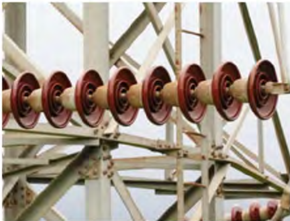
Figure 116 30% rust on caps and insulators are over 50 years old per ETGIS installed date (left). Additional damage could warrant higher priority. Light rust developing with some caps showing signs of dark rust close to 30% of cap (right).
