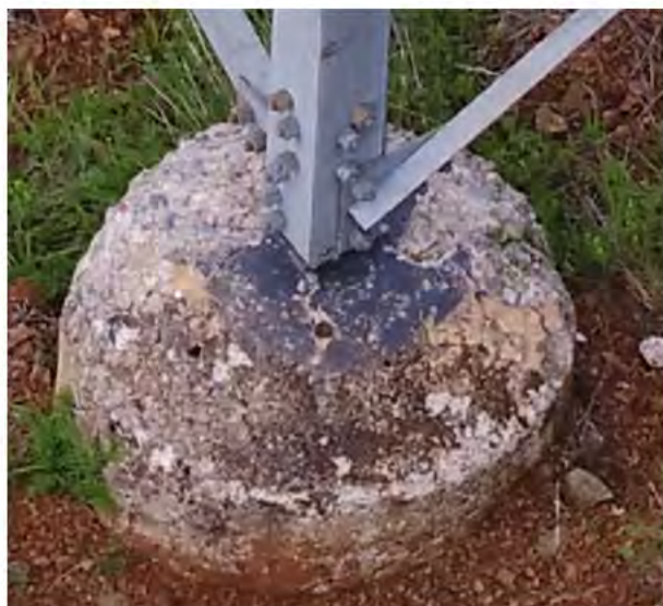
Figure 228 Rebar exposed with > 50% material loss (left). Foundation crack exceeding 1/2" in width AND extended to the stub (right).
