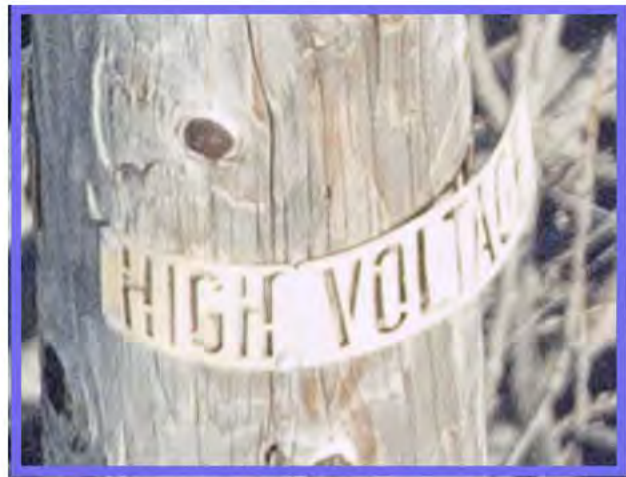
Figure 10 Cracked high voltage sign (left). Damaged sign, no longer legible (right).
