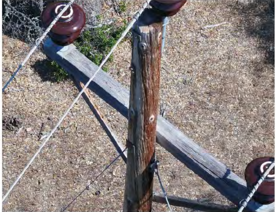
Figure 51 Surface mold (left). Typical pole cracking and shrinking as a result of aging (right).
