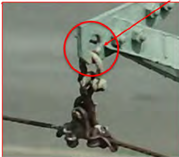
Figure 179 OPGW under anti-climbing guard level, and insulated from structure, public safety risk that requires immediate action. Image on right not grounded at the top of structure.
