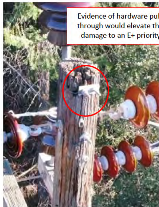
Figure 46 Splitting pole (left). Pole top rot compromising insulator hardware (right).
