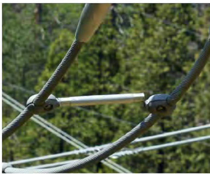
Figure 219 Spacer is tight on the conductor (left). Pre-form style spacers are acceptable as long as they aren't damaged or broken (right).
