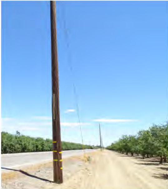
Condition: 1 Priority: No notification required
