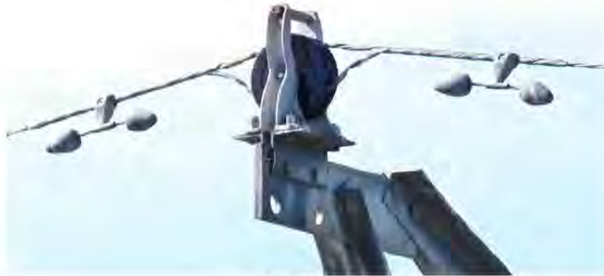
Figure 191 Dampers on shield wire preform are acceptable. Drawing number 102621 for reference.
