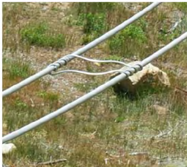
Figure 219 Spacer is tight on the conductor (left). Pre-form style spacers are acceptable as long as they aren't damaged or broken (right).
