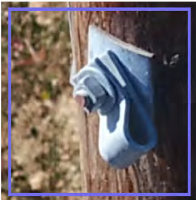
Figure 174 This requires a notification when washers are present on hardware and missing on similar hardware. If washers are missing from all similar hardware, assume that it is per design.
