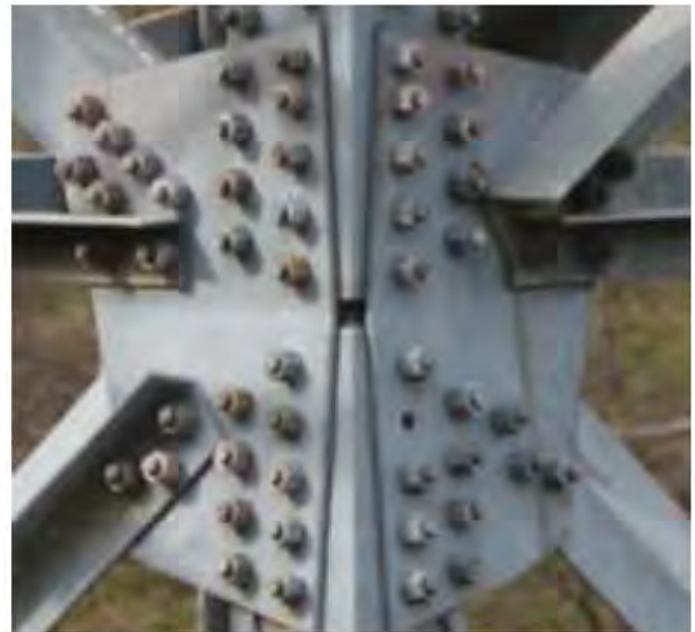
Figure 167 Loose bolt/nut on tower (left). Example of "punched" bolts (right).
