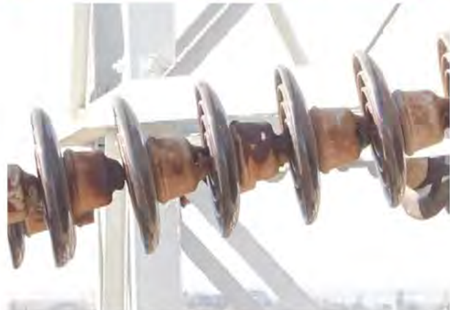
Figure 116 30% rust on caps and insulators are over 50 years old per ETGIS installed date (left). Additional damage could warrant higher priority. Light rust developing with some caps showing signs of dark rust close to 30% of cap (right).
