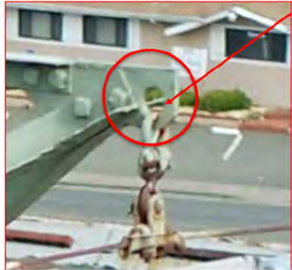
Figure 179 OPGW under anti-climbing guard level, and insulated from structure, public safety risk that requires immediate action. Image on right not grounded at the top of structure.
