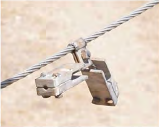
Figure 214 Damper weight in contact with armor rod clamps require a E priority notification (left). If no contact, no tag is necessary (right).
