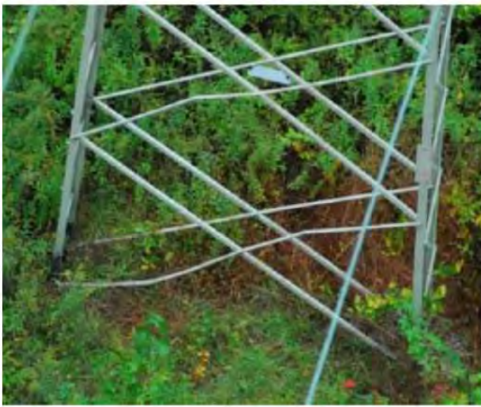
Figure 83 FDA: Structure-Steel|Paint/Coating|Other Lattice tower surface rust (left). FDA: Structure-Tower|No Good/ Out of Stdrd |Repair Bent primary member on crossarm (right). Any additional bent members on the same crossarm should be considered a possible A priority.
