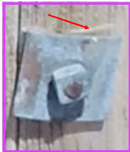
Figure 174 This requires a notification when washers are present on hardware and missing on similar hardware. If washers are missing from all similar hardware, assume that it is per design.
