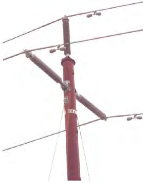
Condition: 1 Priority: No notification required
