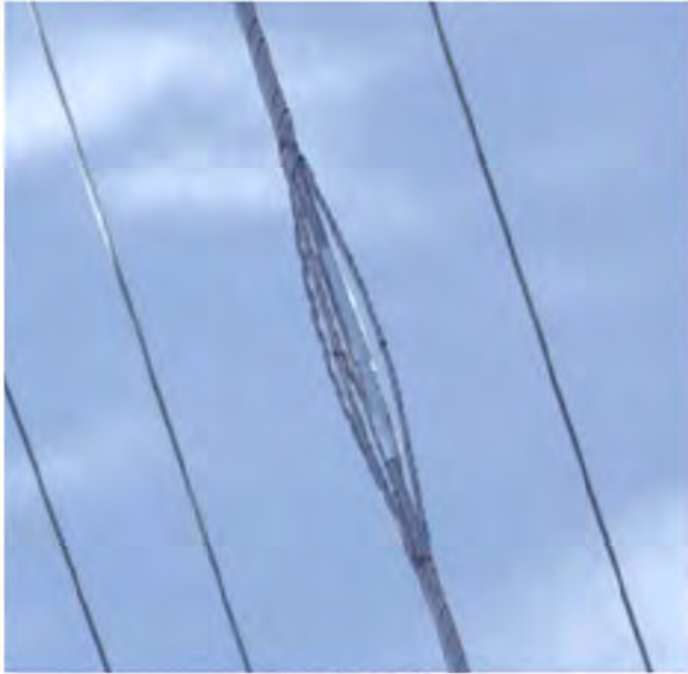
Condition: 1 Priority: No notification required
