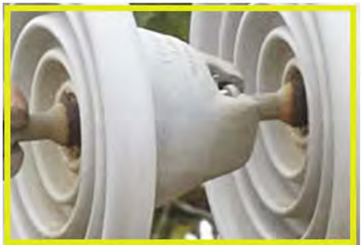
Figure 118 Example of rusted insulator pins (left) that also has a loose cotter key. Example of emergency level rusted insulator pins (right).
