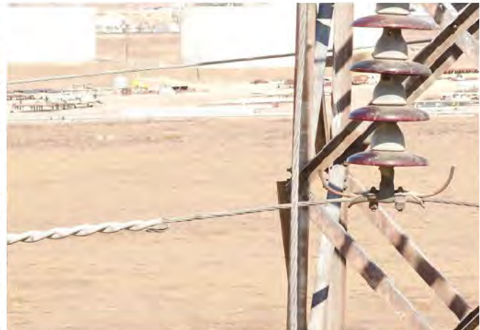
Figure 221 Failed splice (left). Splice is not compressed on one side (right).
