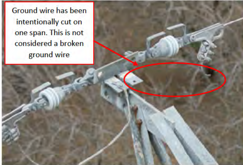
Figure 181 Overhead ground/shield wire
