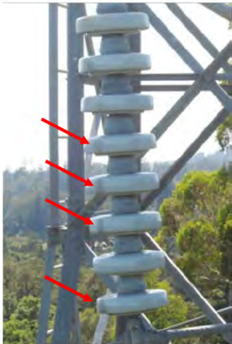
Figure 114 Example of tracking visible on insulator caps (left). Right image shows minor contamination, which due to the orientation of the string and the flow of water, resembles tracking. Because this is contamination and not damage, no tag is necessary. Tracking is generally wider and doesn't occur in such a straight and uniform line.
