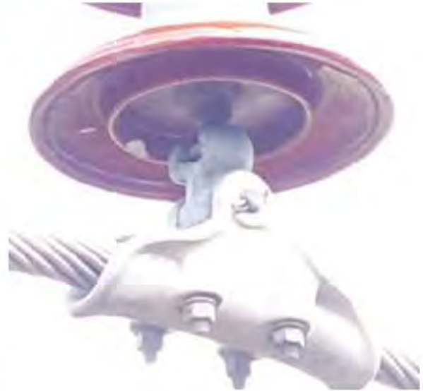
Figure 110 Insulators with chipped bells larger the 1-1/2 inches in diameter.
