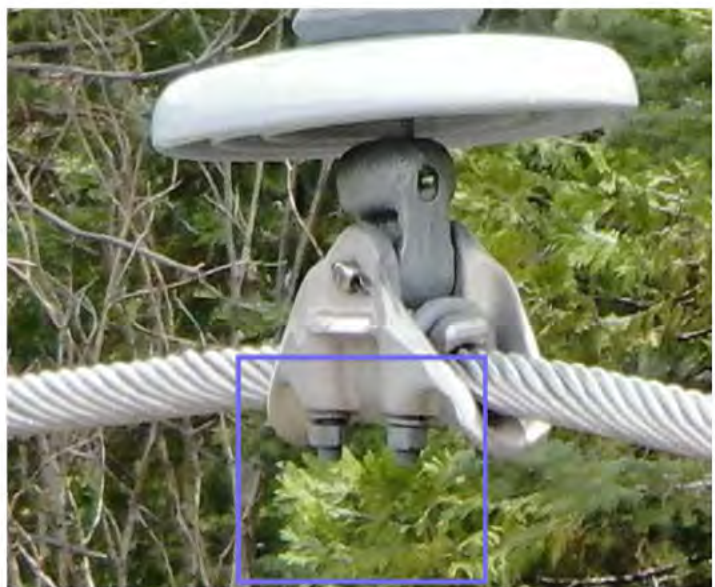
Figure 145 J-bolts may appear on the outside of the washer/nut, but tight on the inside, closest to the conductor (see above). These nuts cannot be tightened any further and should be considered tight. No tags required, even if the lock washer isn't completely compressed because of this space.
