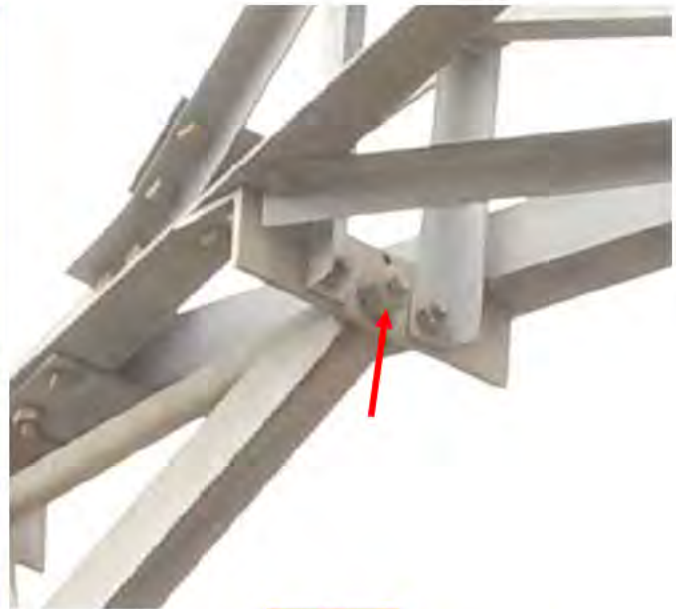
Figure 165 Washer is missing between the swing plate and the cotter key. If the cotter key is damaged or worn, the hardware and conductor can fall. The "Steel" FDA should be used if this takes place on a tower or on a steel pole
