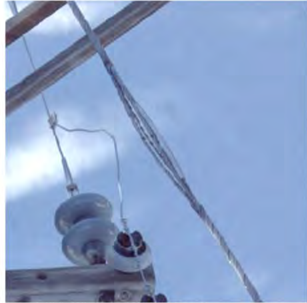
Condition: 1 Priority: No notification required
