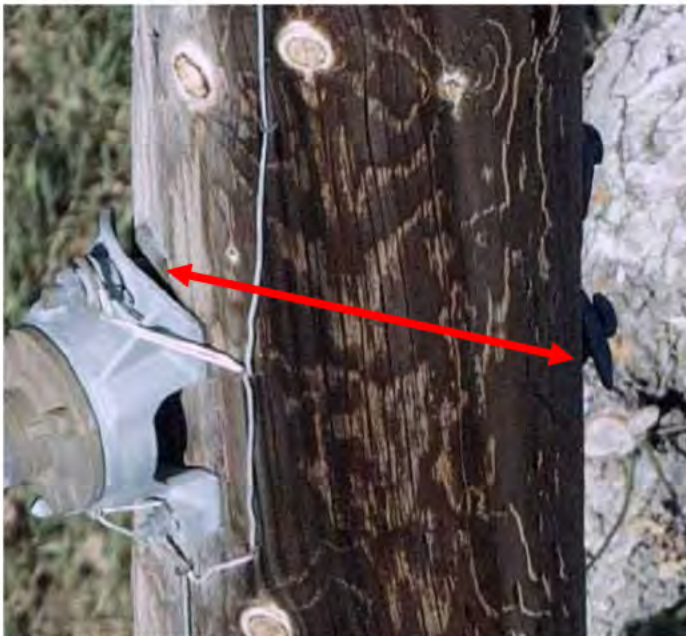
Figure 176 Loose U-bolt holding the insulator to the pole (left). Loose sister eye (right).
