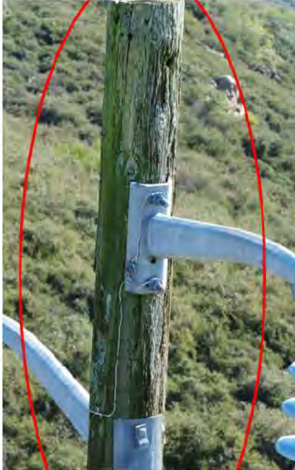
Figure 51 Surface mold (left). Typical pole cracking and shrinking as a result of aging (right).
