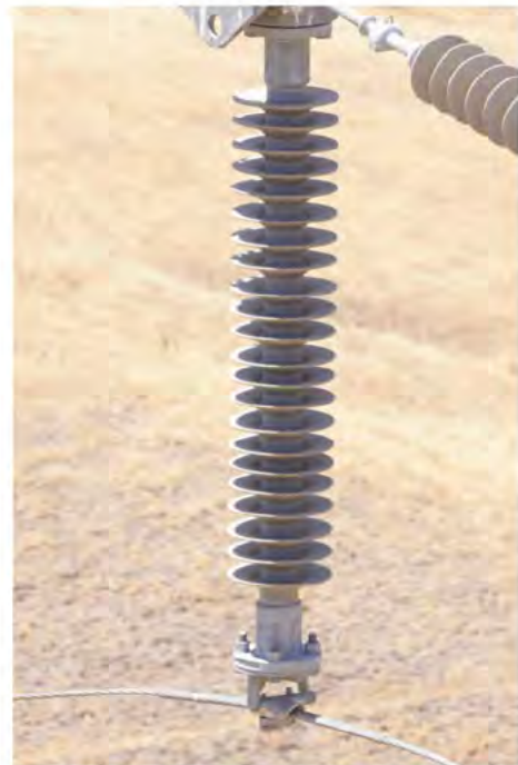
Figure 155 Automatic dead-end shoes which should be removed when found.
