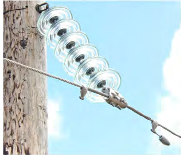
Figure 214 Damper weight in contact with armor rod clamps require a E priority notification (left). If no contact, no tag is necessary (right).
