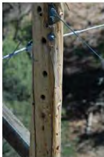
Pole cracks/rot with material loss (left). Single pole deflection on H-frame (right).
