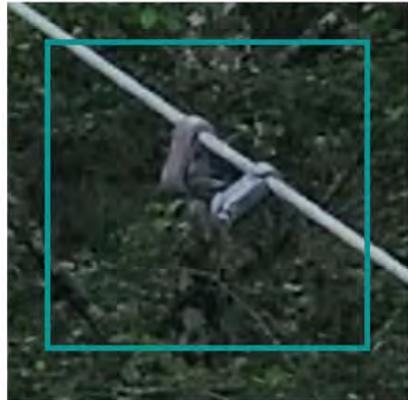
Figure 203 Examples of damaged conductor, 1 strand to 5%. Broken strands up to 5% is an F priority.
