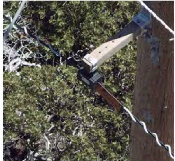
Figure 198 ADSS twisted at hardware attachment, and armor/reinforcement rod out of position (left). Missing reinforcement rod on ADSS, which requires repair (right).
