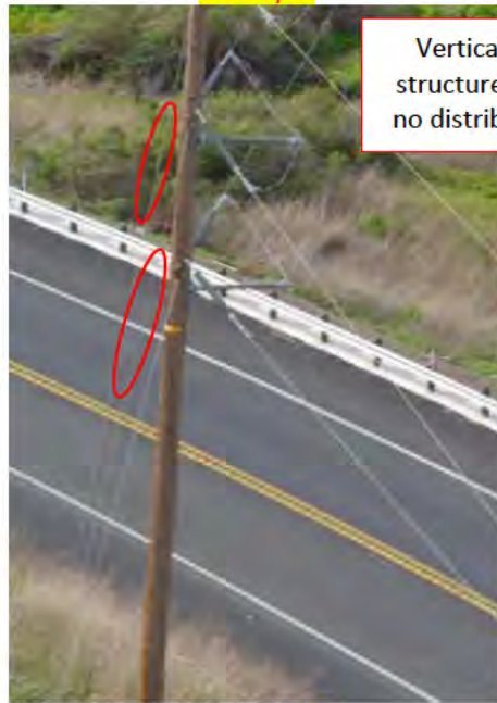
Figure 23 Examples of guyed structures with missing fiberglass rod. If congestion exists at Transmission-level, assign E-priority.
