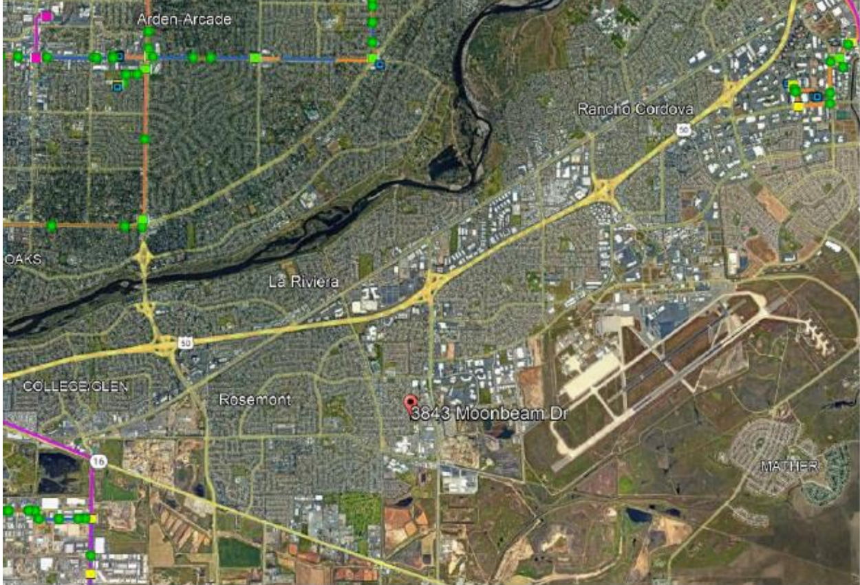
Photo 4: Photo of facility mapping provided by operator Astound/Wave Broadband.
