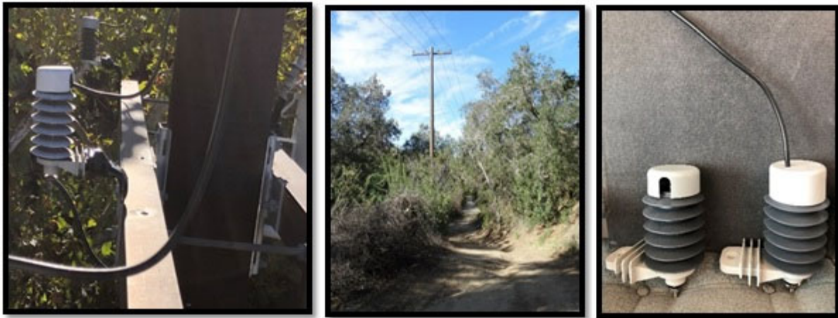
Figure 15: (a) Concealed Lightning Arrester (b) Ductile Iron Pole (c) Comparison of Lightning Arrester Models
