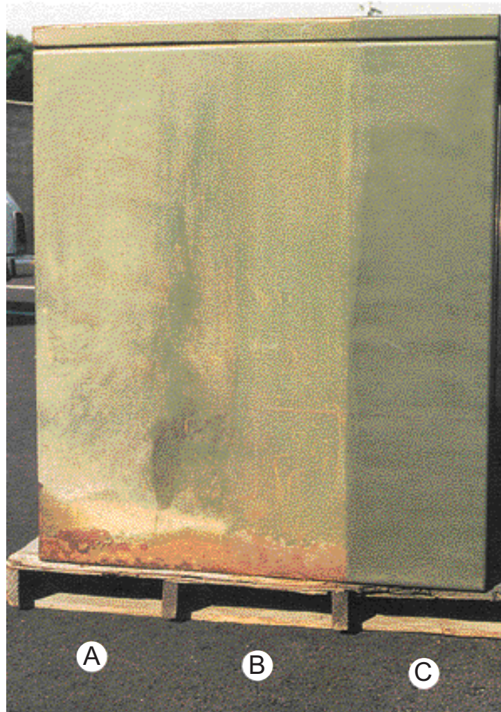
Figure 7-9: Field Painting of Pad-Mounted Equipment (9 of 12)
