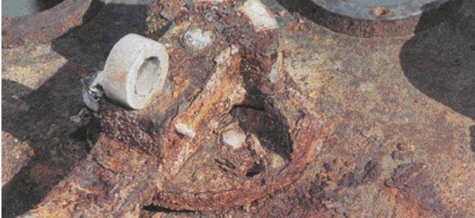
Figure 5–14: Maintenance and Refurbishing — Example 2 of 4
