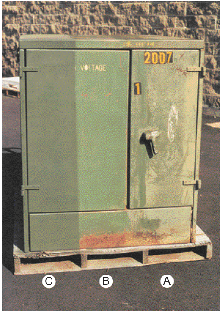
Figure 7-1: Field Painting of Pad-Mounted Equipment (1 of 12)
