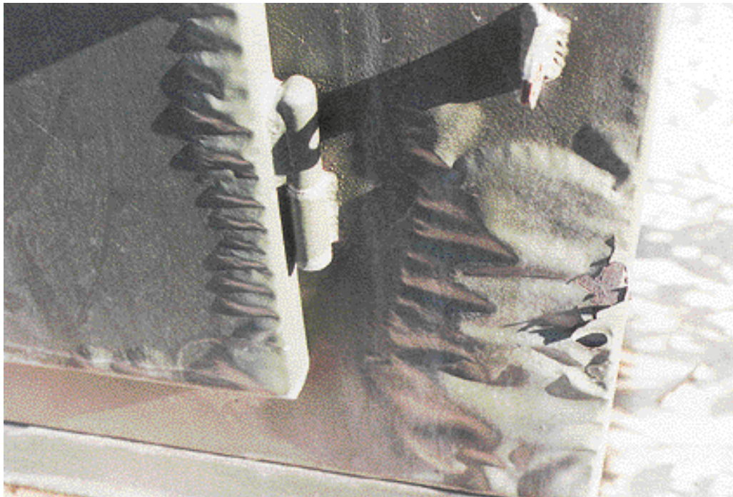
Figure 6–13: Significant Blistering of Paint
