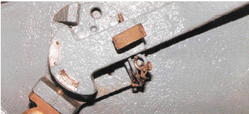
Figure 5–16: Maintenance and Refurbishing — Example 4 of 4
