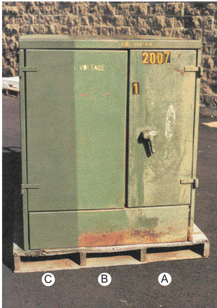
Figure 7-1: Field Painting of Pad-Mounted Equipment (1 of 12)
