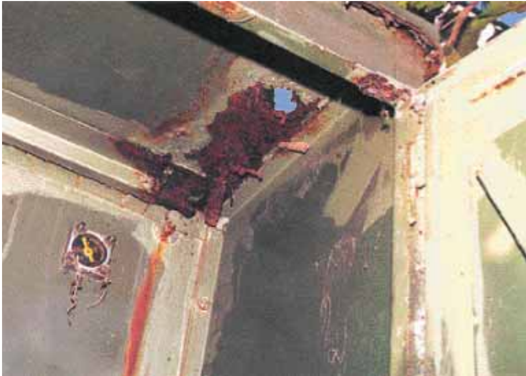
Figure 6–1: Opening Completely Through the Enclosure Wall
