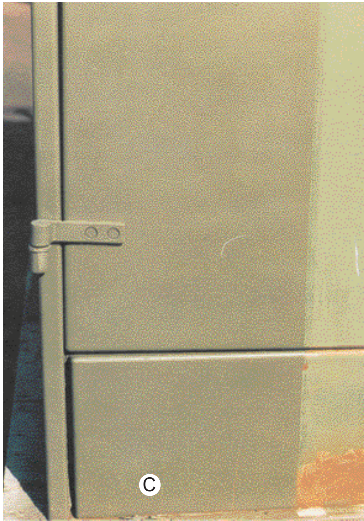
Figure 7-12: Field Painting of Pad-Mounted Equipment (12 of 12)
