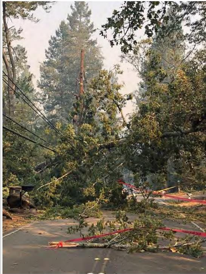
Fig. 65. Example of damage to electric lines from fallen tree
