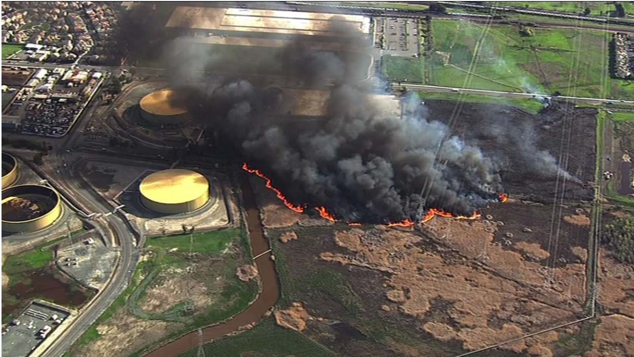
Figure TBC 10- 1. Smoke from Small Brush Fire Near the Converter Station in March 2019 (Copyright © 2019 KGO-TV) #3
