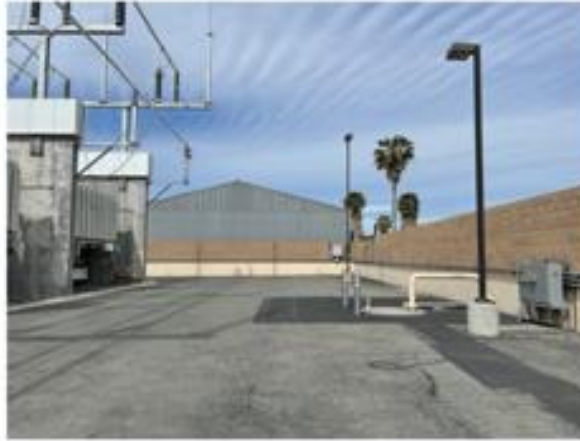
Figure TBC 8.1.2- 3. Hardscaped AC yard
