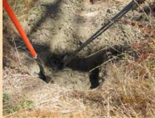
After: Vegetation cleared from anchor
