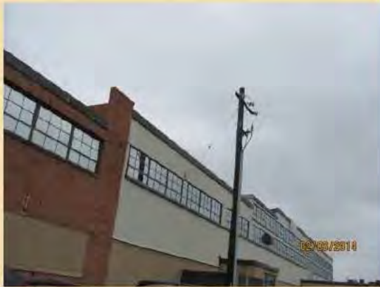
At this Location: Acceptable down guy attached to building, no marker required.
