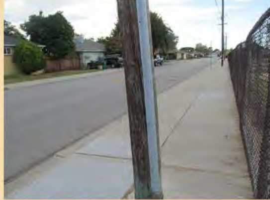
After: 1.5 inch u-shaped molding installed over existing wood molding
