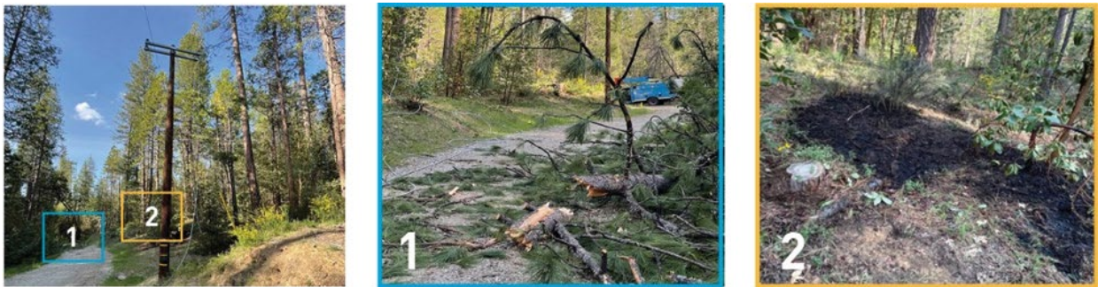
Figure 3 PG&E Covered Conductor Effectiveness – Example 2
