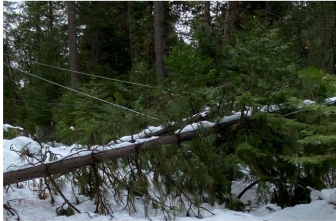
Figure 4 PG&E Covered Conductor Effectiveness – Example 3
