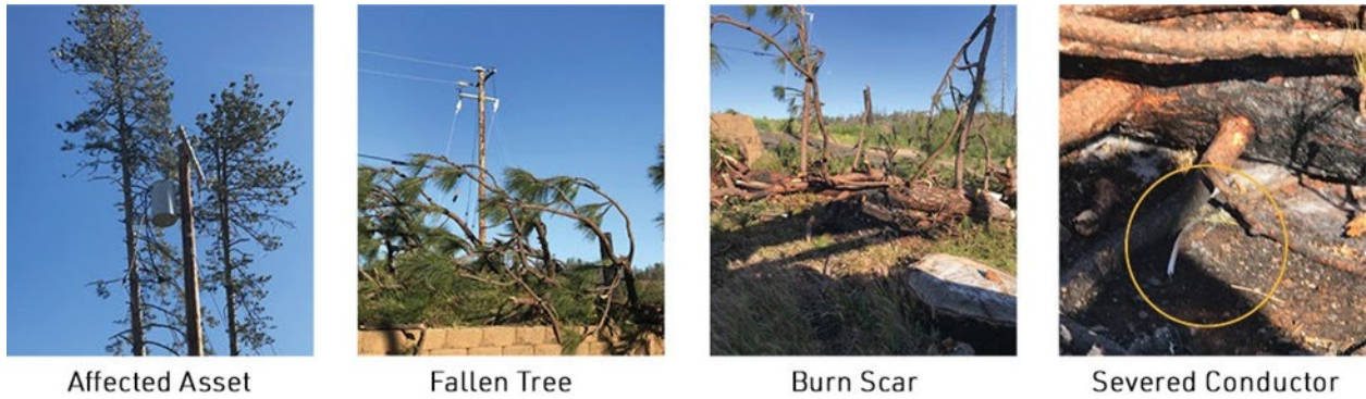
Figure 2 PG&E Covered Conductor Effectiveness – Example 1
