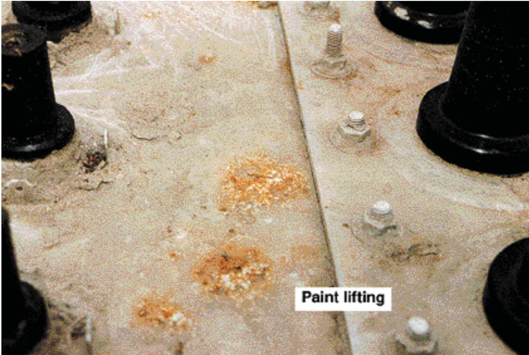
**Figure 5-12: Light Corrosion — Example 3 of 3**
