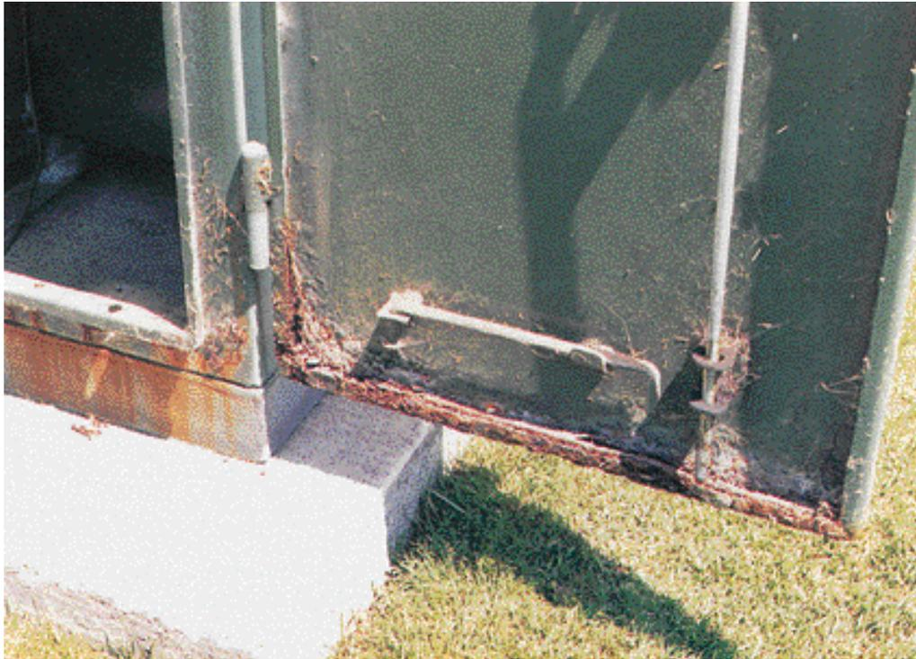
Figure 6–20: Peeling of Paint with Moderate Pitting
