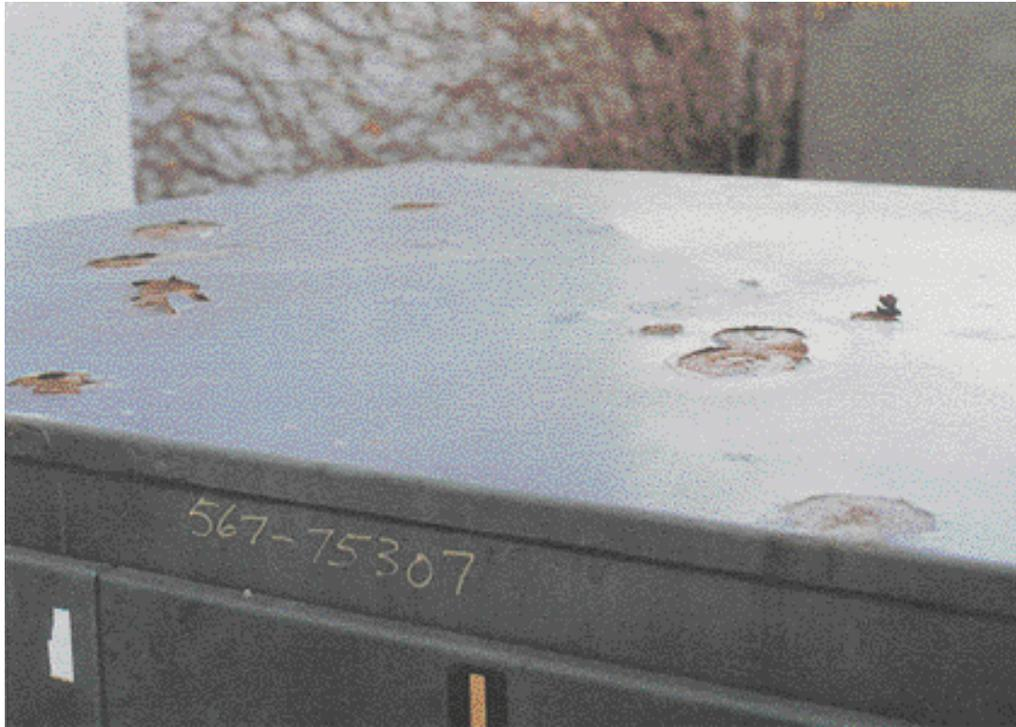
**Figure 6-18: Moderate Corrosion with Significant Loss of Paint at Base**
