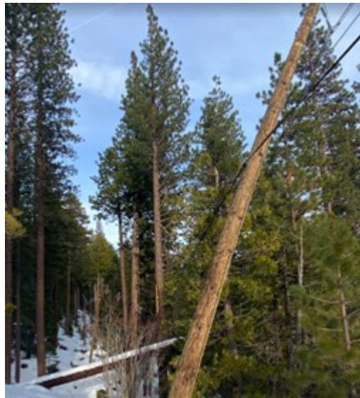
Figure CC-7 Liberty Spacer Cable System Preventing a Fault – Viewpoint 2
