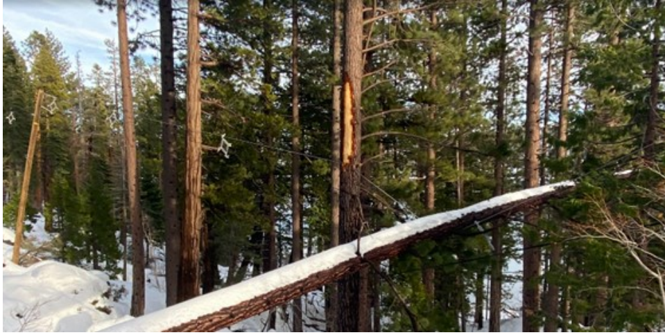
Figure CC-7 Liberty Spacer Cable System Preventing a Fault – Viewpoint 2
