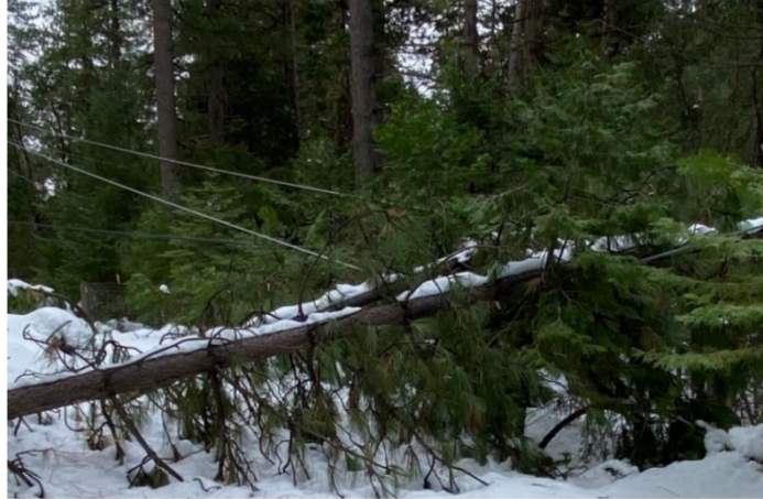
Figure CC-4 PG&E Covered Conductor Effectiveness – Example 3
