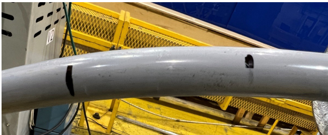
Figure 6-26: Sample 3K.1.1 - 17 kV, 1/0 AWG ACSR Condition after Test
