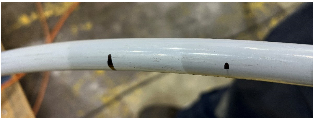
Figure 6-30: Sample 3K.1.3 - 17 kV, 1/0 AWG ACSR Condition after Test
