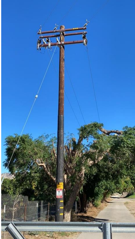
Item13G1mg1: Overall pole
