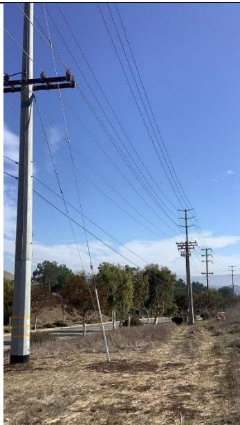
Item3GImg3: Vegetation cleared
