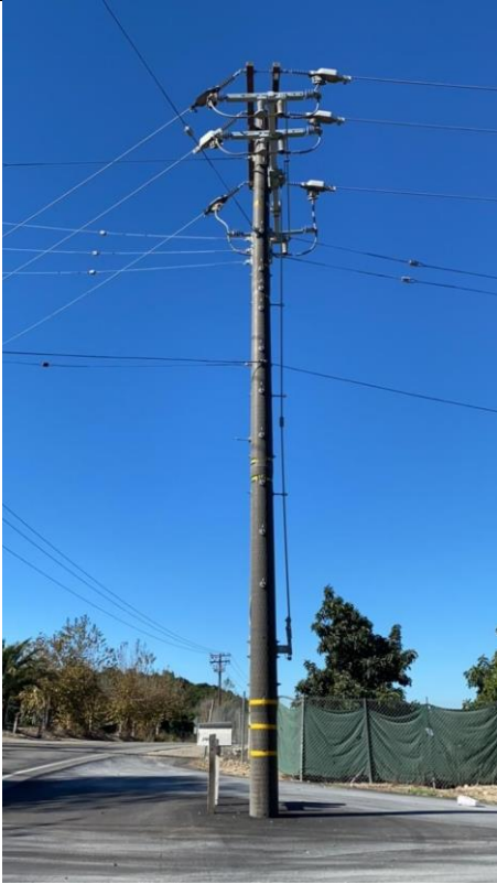
Item6GImg1: Overall pole
