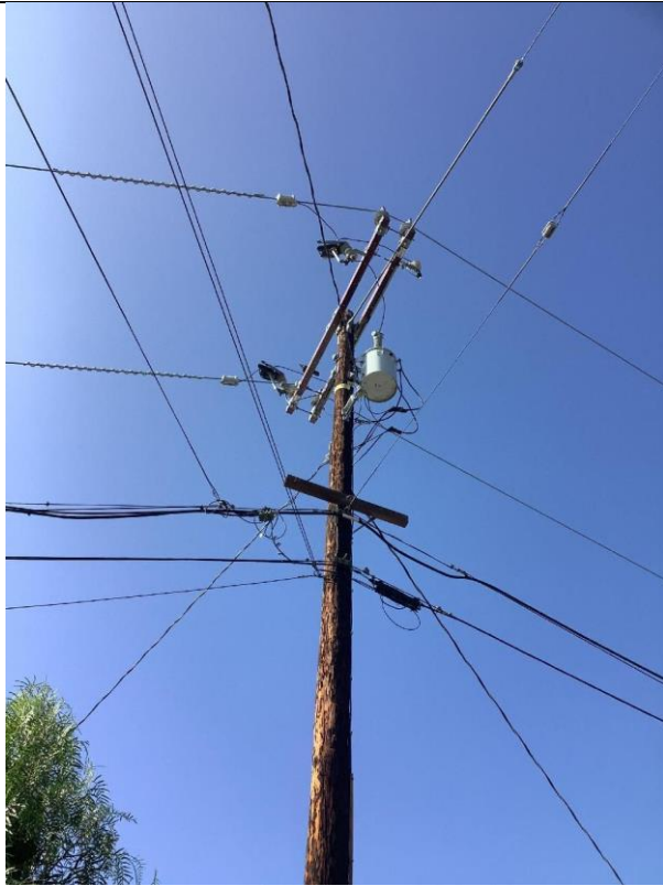
Item8GImg1: Overall pole
