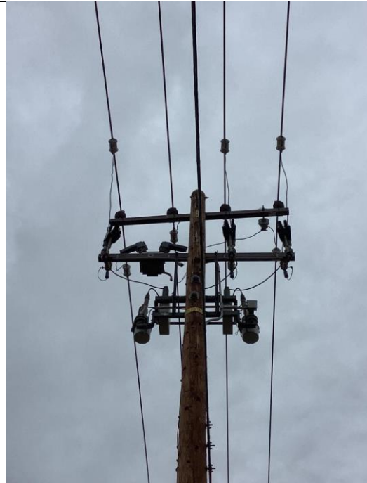
Item13G1mg2: Overall pole
