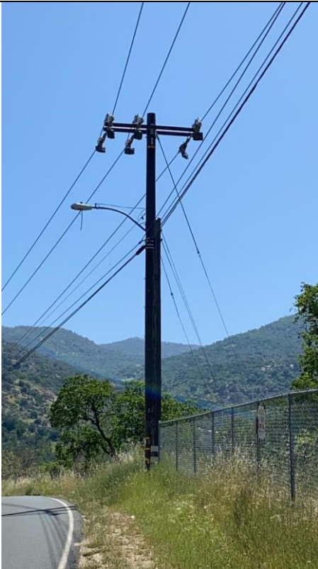
Item8GImg1: Overall pole
