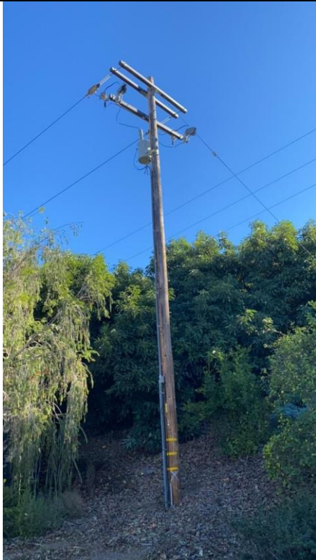
Item12GImg1: Overall pole
