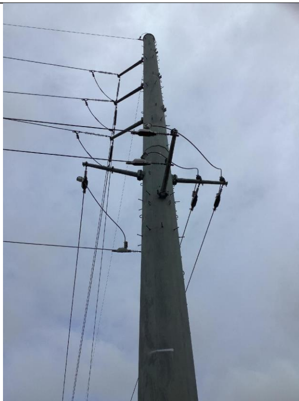
Item20Gimg2: Overall pole
