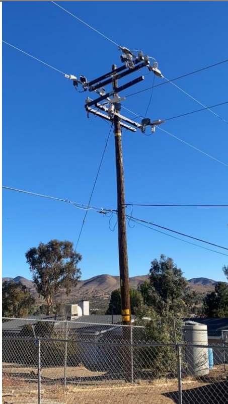
Item6GImg1: Overall pole
