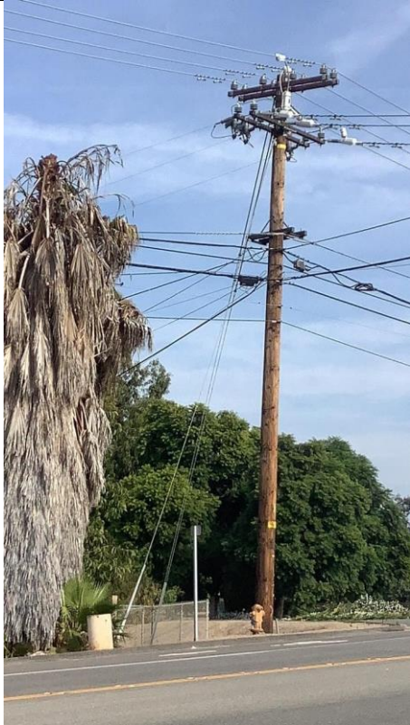
Item6GImg1: Overall pole
