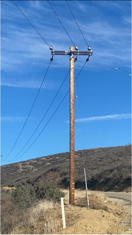
Item9GImg1: Overall pole
