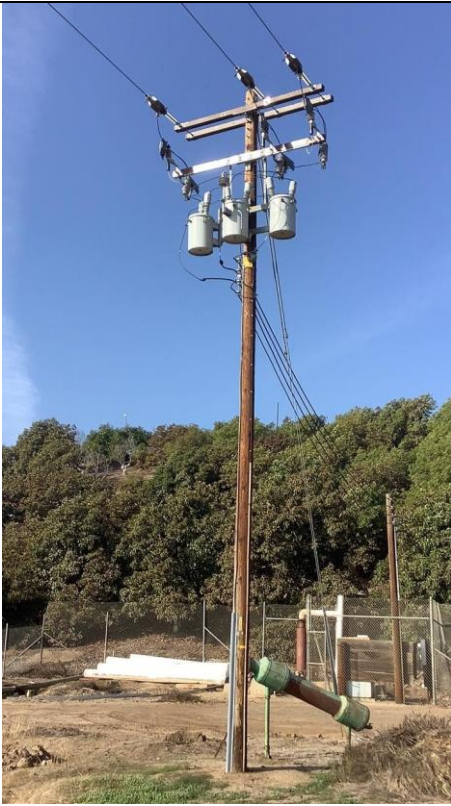
Item13GImg1: Overall pole
