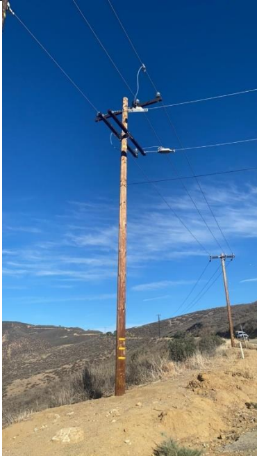
Item8GImg1: Overall pole
