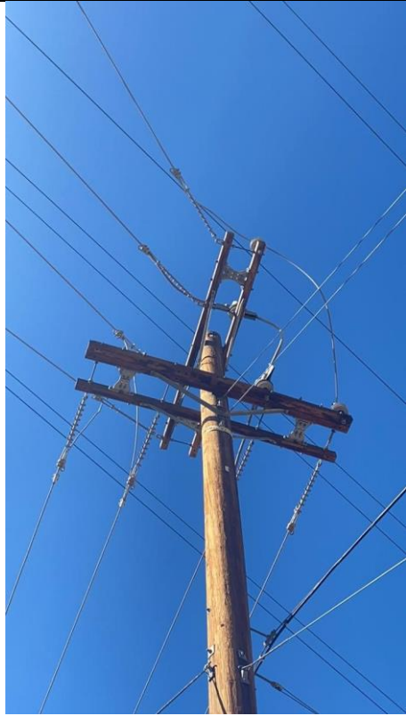
Item15IA1Img2: Overall pole
