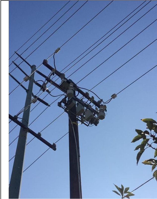
Item4GImg1: Overall pole
