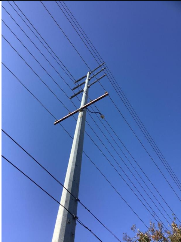
Item2GImg1: Overall pole
