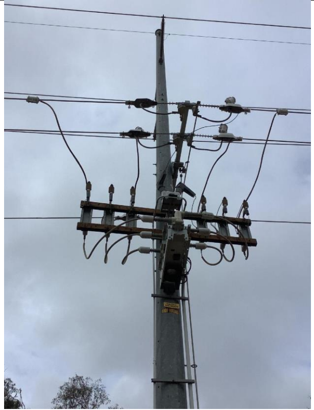
Item19G1mg2: Overall pole
