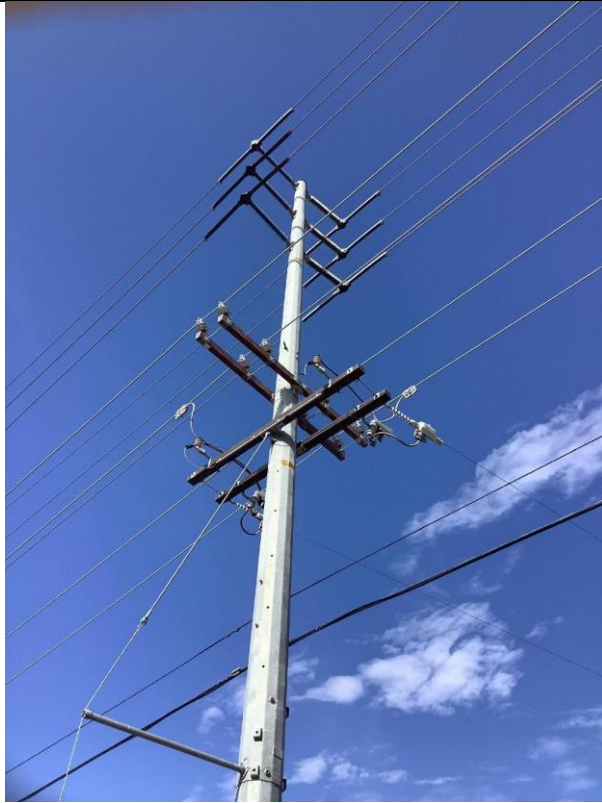
Item6GImg1: Overall pole
