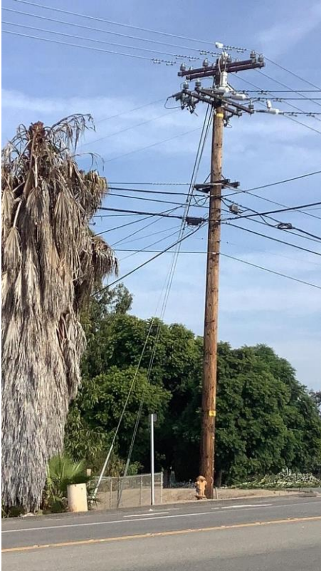
Item6GImg1: Overall pole
