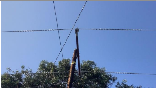
Item10IA1Img1: Overall crossarm
