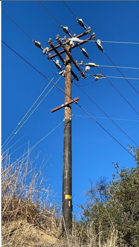
Item1Gimg1: Overall pole
