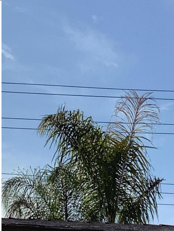
Item9IA1Img3: Palm fronds contacting conductor
