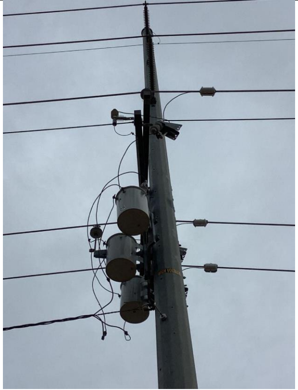
Item18G1mg2: Overall pole
