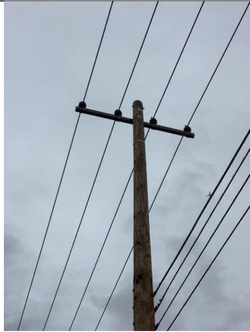
Item12GImg2: Overall pole
