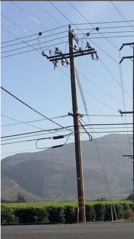
Item14G1mg1: Overall pole
