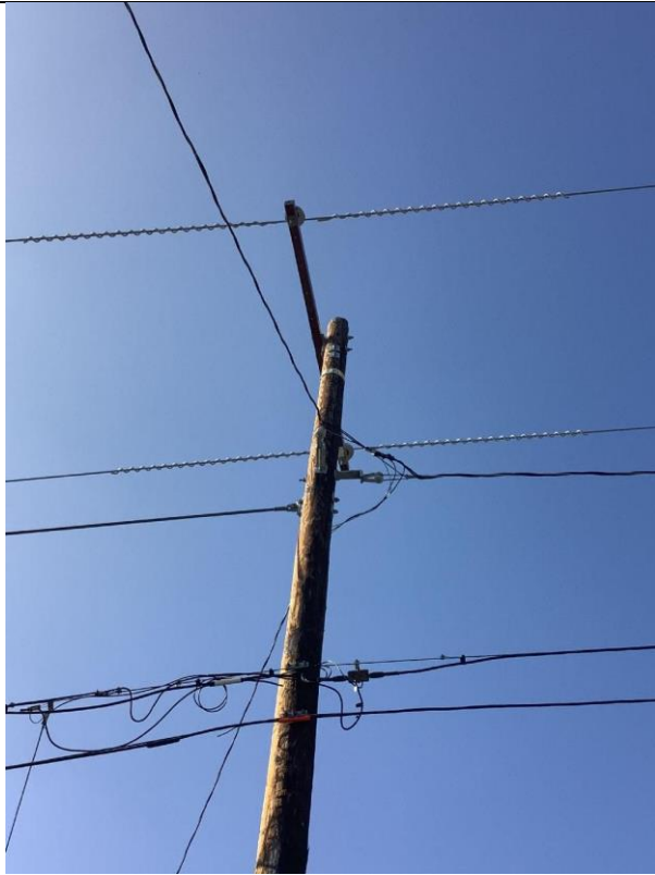
Item9GImg1: Overall pole
