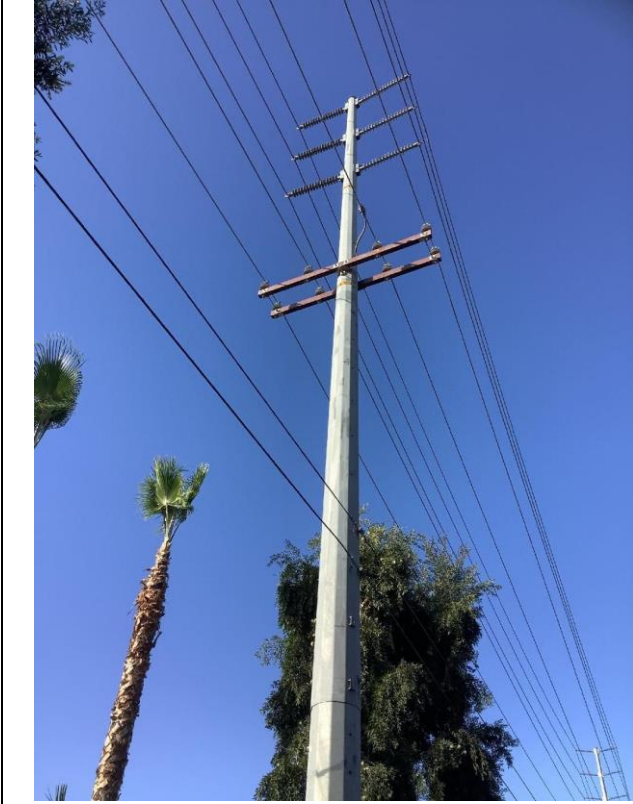
Item1G1mg1: Overall pole
