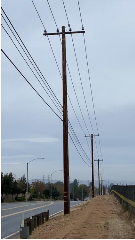
Item6GImg1: Overall pole
