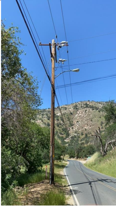
Item7GImg1: Overall pole
