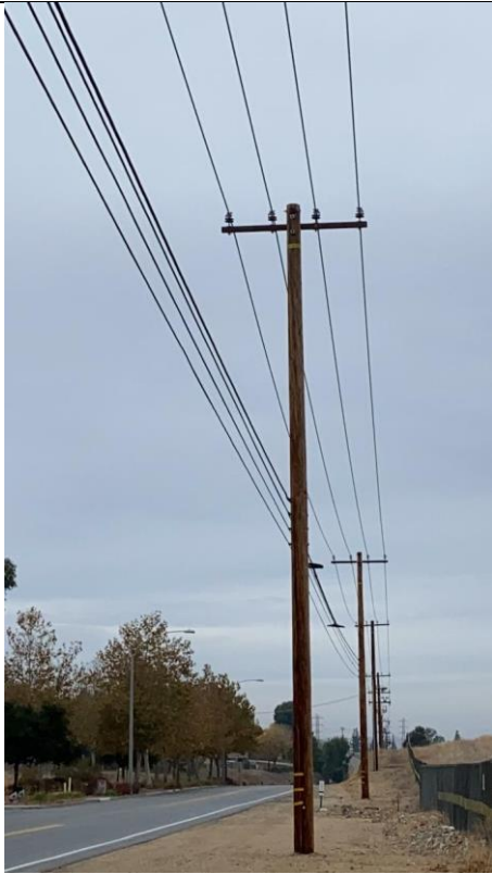
Item10GImg1: Overall pole
