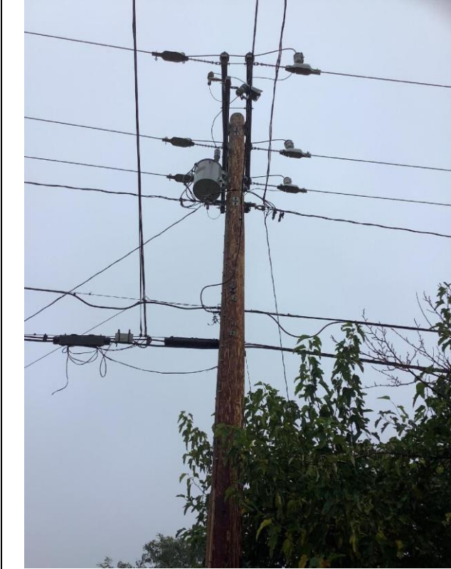
Item1Gimg1: Overall pole
