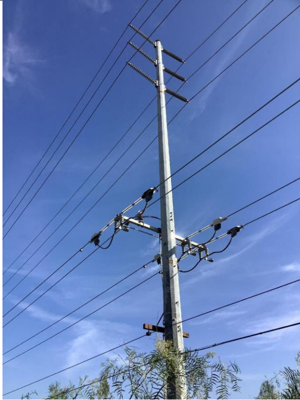
Item13GImg1: Overall pole
