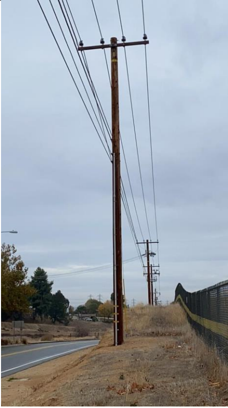
Item11GImg1: Overall pole
