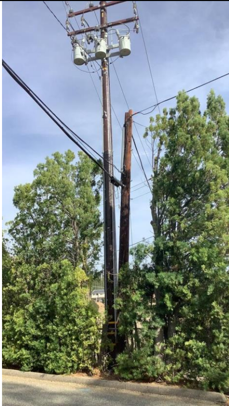
Item7GImg1: Overall pole
