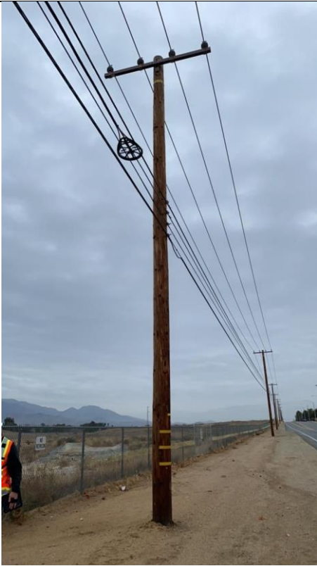
Item9GImg1: Overall pole
