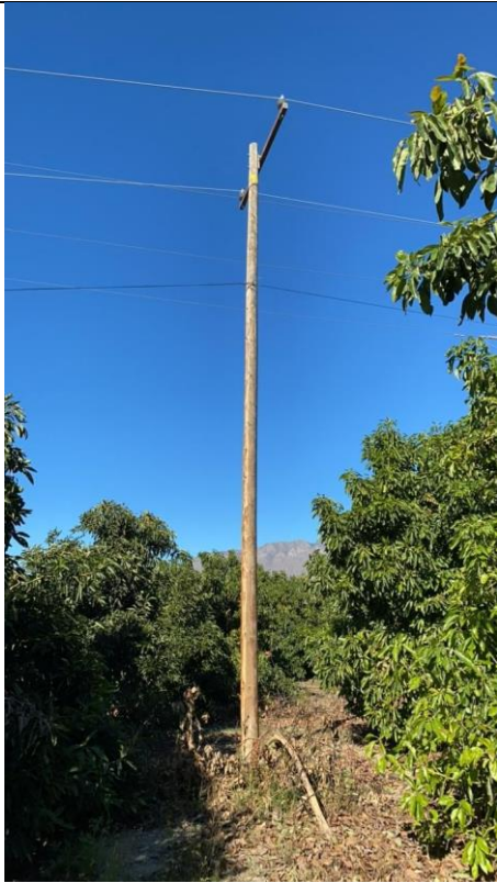
Item9GImg1: Overall pole
