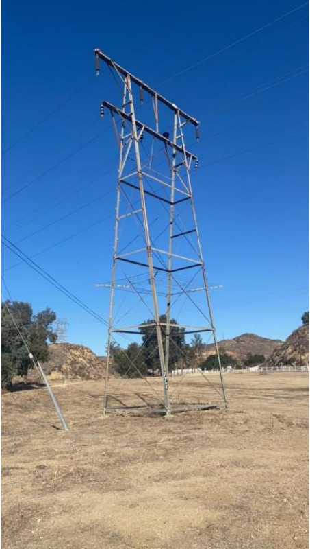
Item17GImg1: Overall structure
