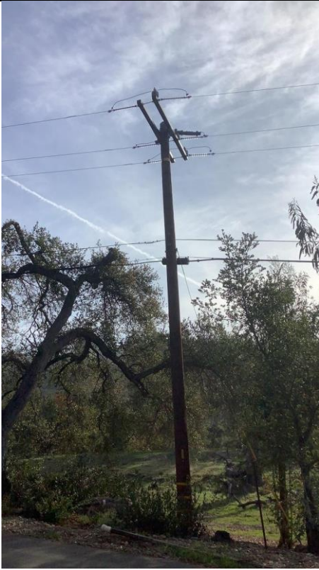
Item1Gimg1: Overall Pole
