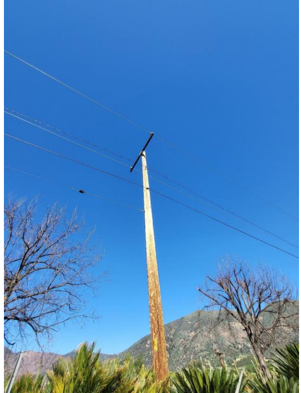
Item2Gimg2: Overall Pole
