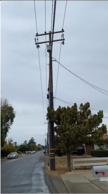
Item15GImg1: Overall pole
