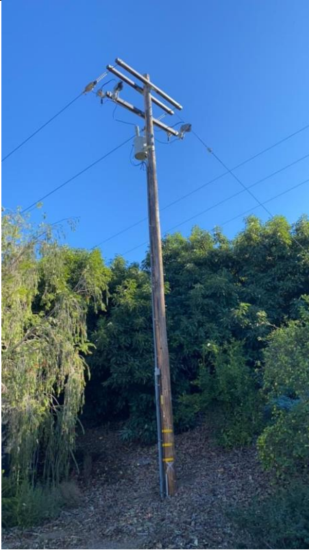
Item12GImg1: Overall pole
