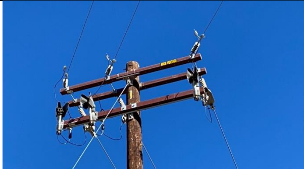
Item13IA1mg1: Bare wire to covered conductor
