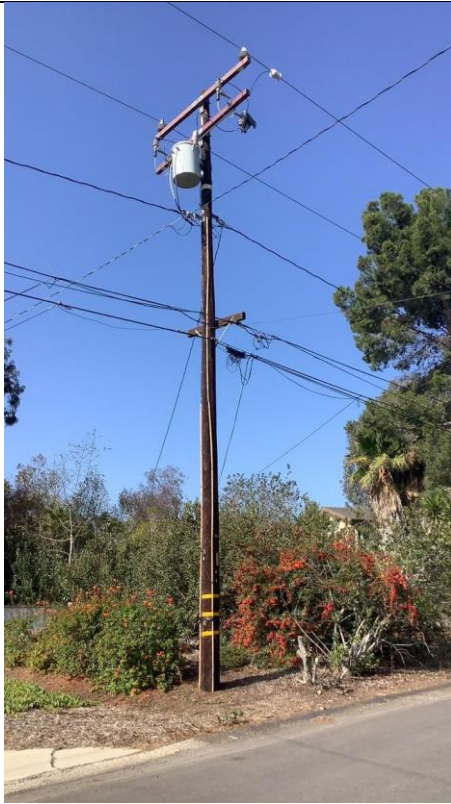
Item11GImg1: Overall pole
