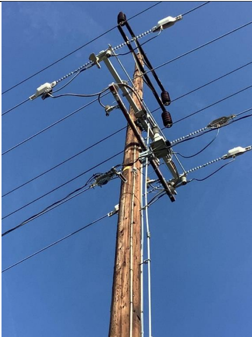
Item11G1mg1: Overall pole
