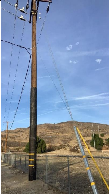
Item11IA1Img1: Overall view of down guy
