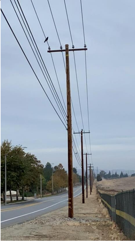
Item8GImg1: Overall pole
