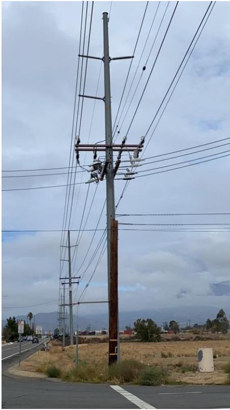
Item16G1mg1: Overall pole
