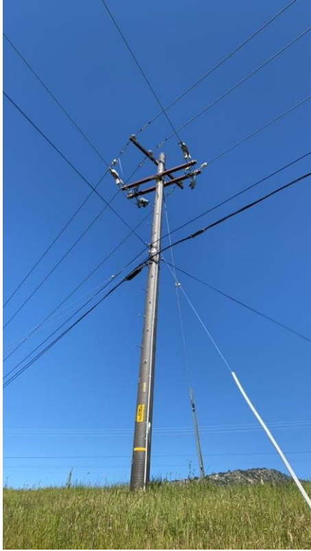
Item4GImg1: Overall pole
