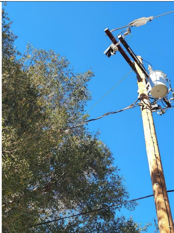
Item1GImg2: Overall Pole
