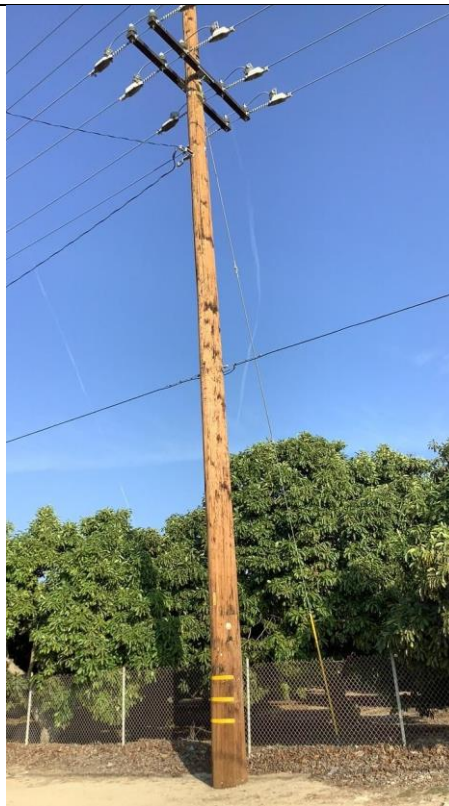
Item1Gimg2: Overall view of the pole, covered conductor installed
