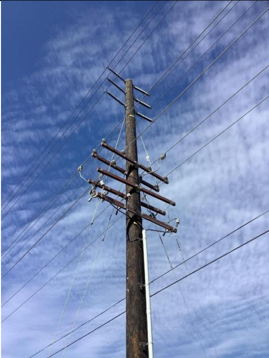
Item5GImg1: Overall pole
