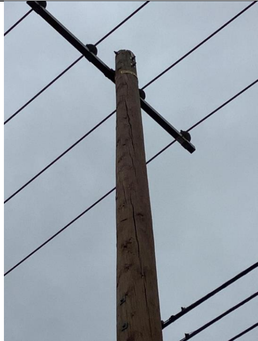
Item7GImg2: Overall pole
