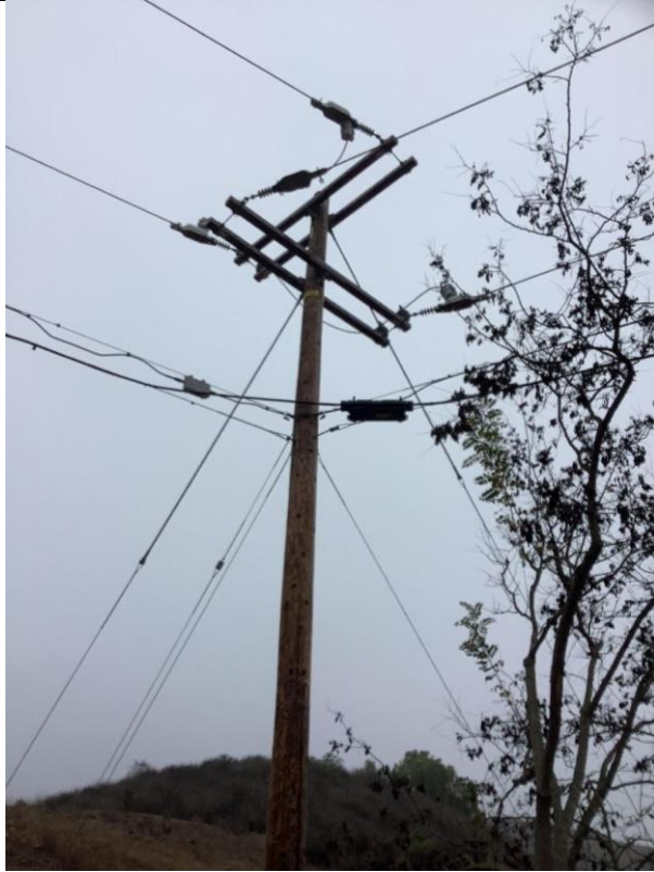
Item4GImg1: Overall pole
