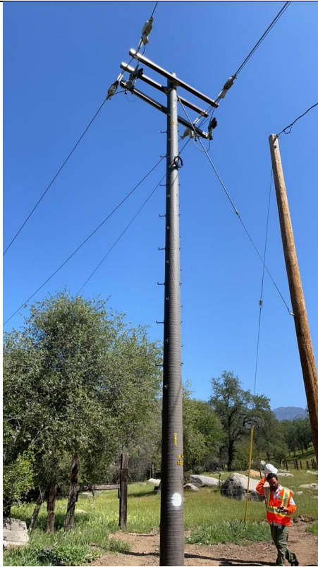
Item2GImg1: Overall pole
