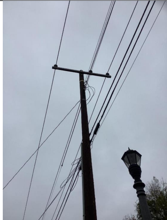
Item14GImg2: Overall pole
