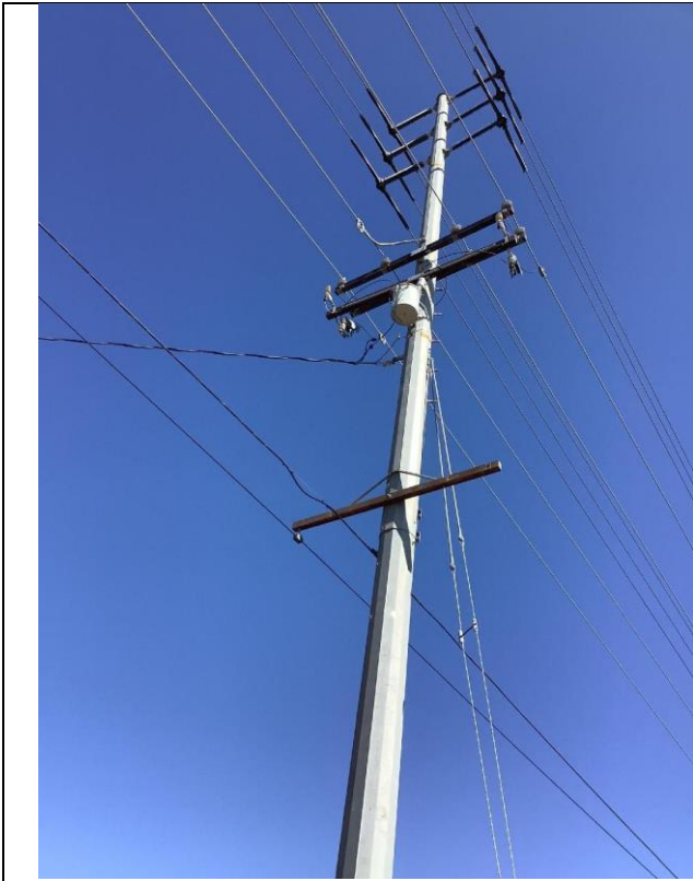
Item9GImg1: Overall pole
