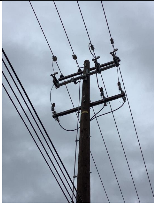
Item11G1mg2: Overall pole
