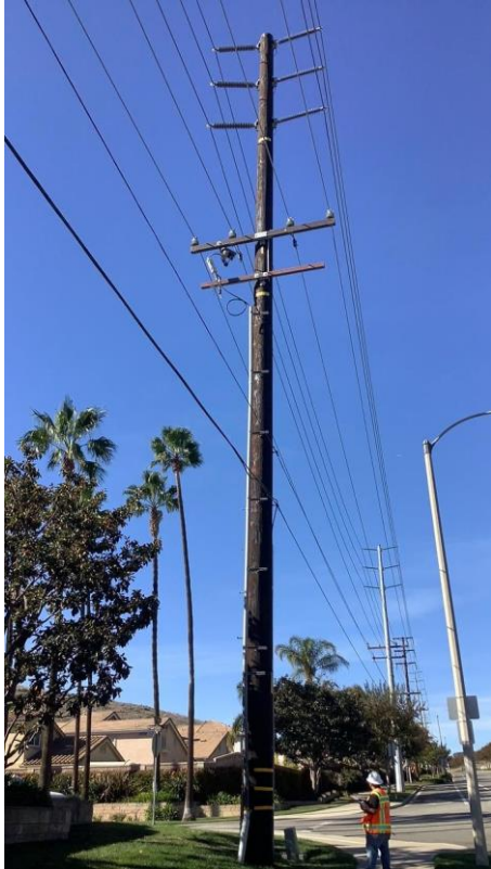
Item5GImg1: Overall view of pole
