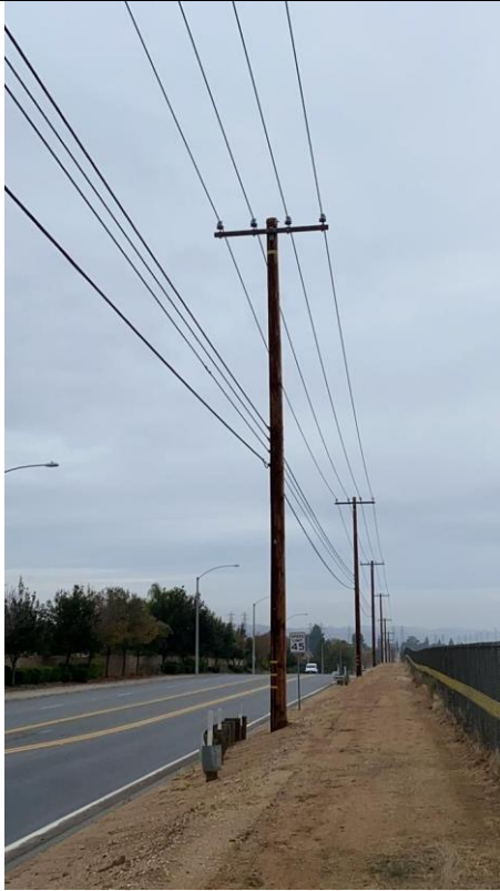
Item5Gimg1: Overall pole
