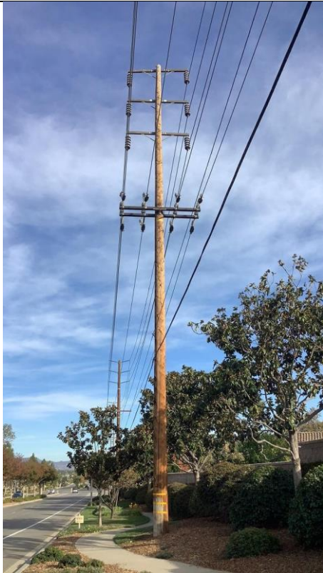
Item3GImg1: Overall pole
