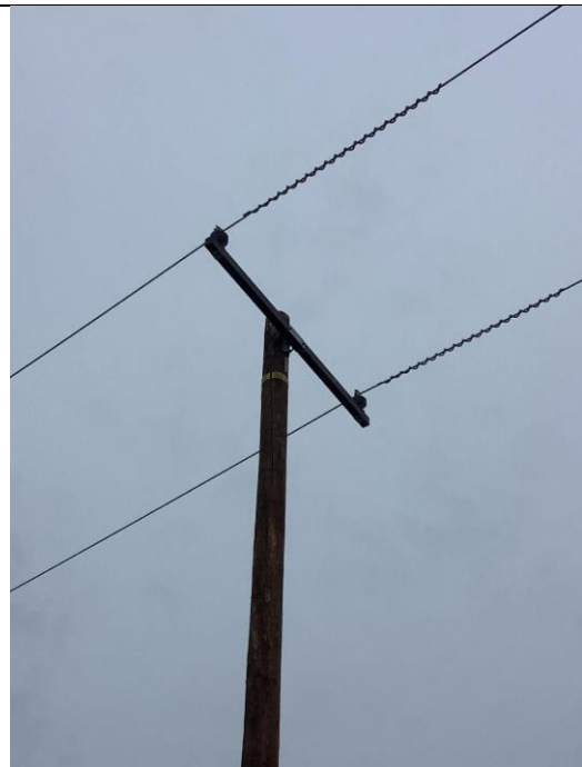
Item3GImg2: Overall pole
