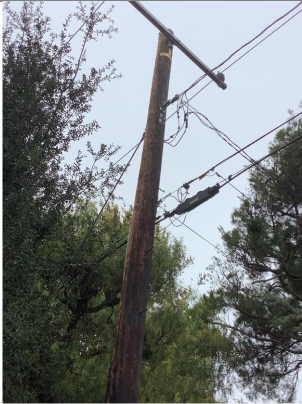
Item6GImg1: Overall pole
