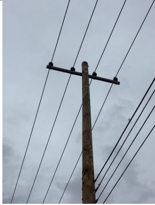
Item12GImg2: Overall pole
