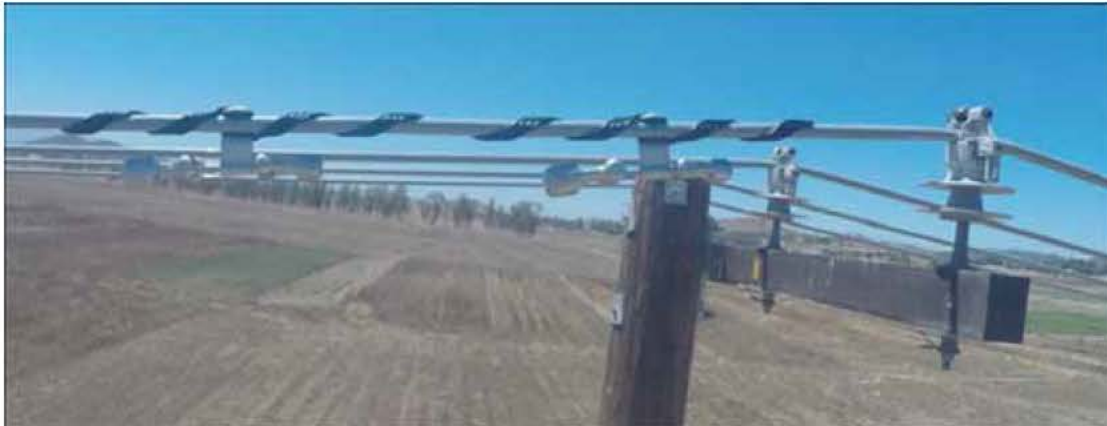
Figure CC 190–13: Installed Spiral Rod Stockbridge Damper
