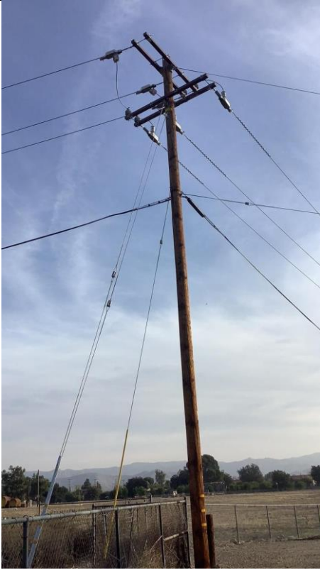
Item9GImg1: Overall pole
