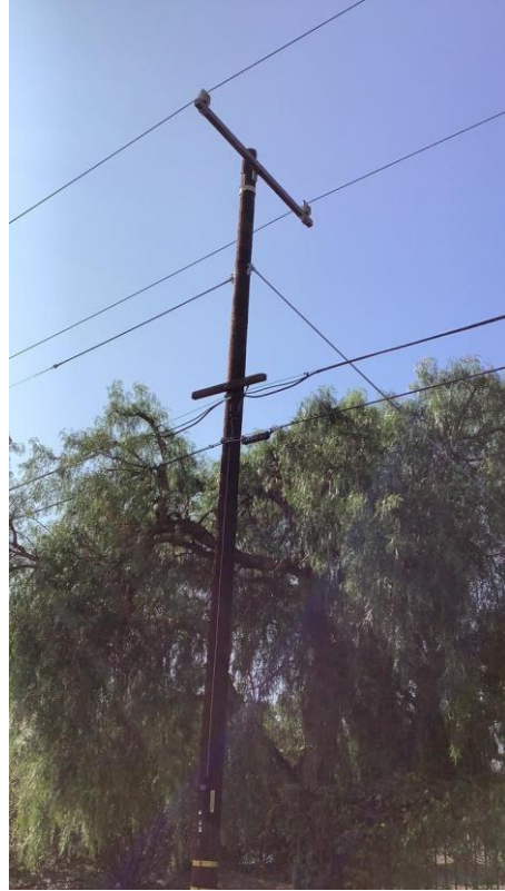
Item1Gimg2: Overall view of the pole and covered conductor installation
