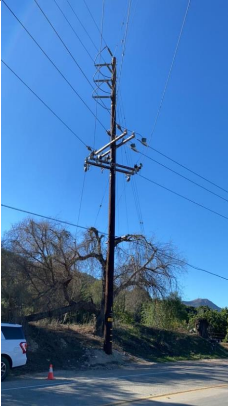
Item7GImg1: Overall pole
