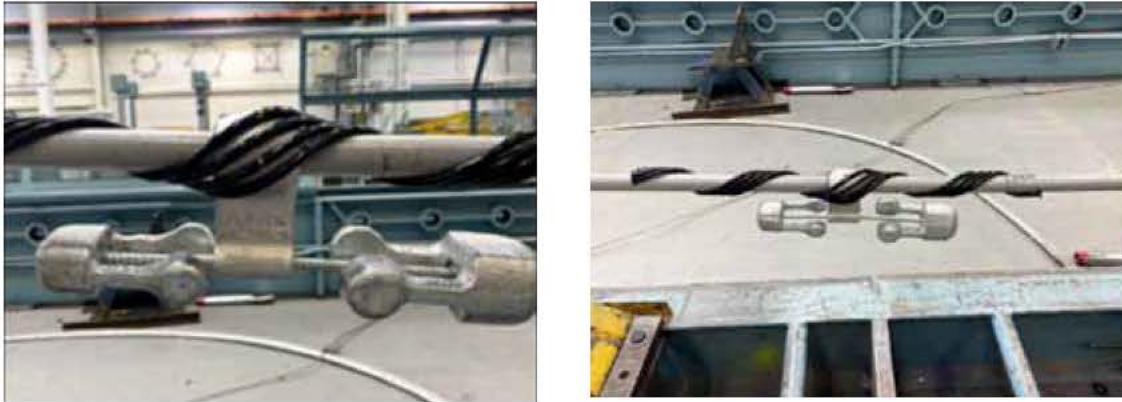
Figure CC 190–12: Completed Attachment Rod Placement
