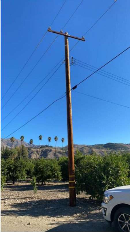
Item3GImg1: Overall pole
