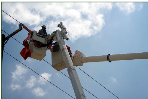
Shown: Utility Workers Using Bucket Trucks
