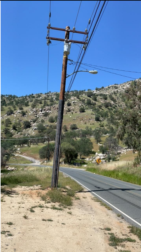
Item5GImg1: Overall pole
