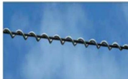
Figure 2: Spiral Damper
