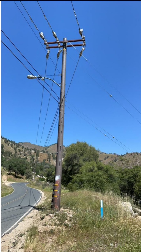
Item6GImg1: Overall pole
