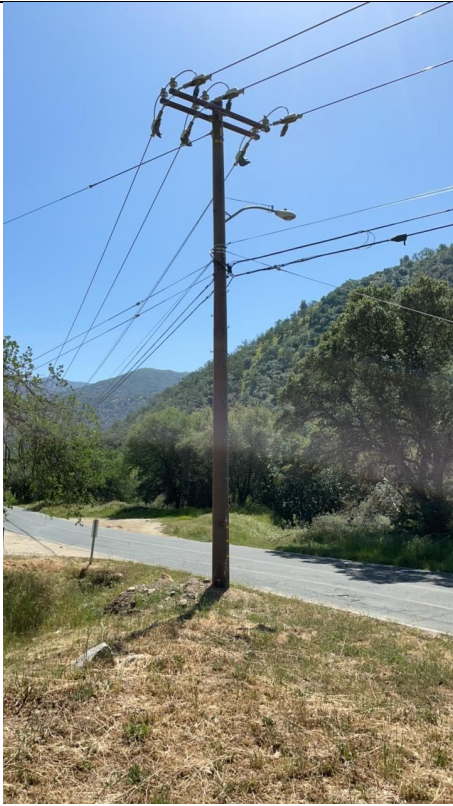
Item4GImg1: Overall pole
