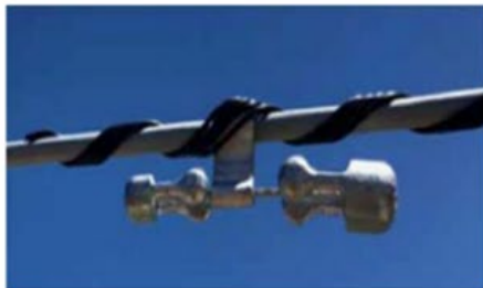
Figure 1: Stockbridge Damper
