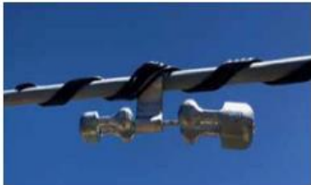
Figure 1: Stockbridge Damper
