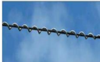
Figure 2: Spiral Damper
