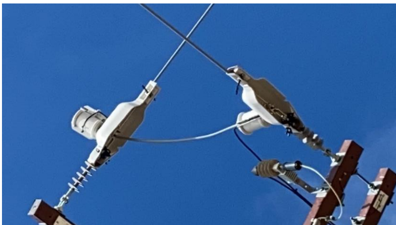
Item8IA1Img1: Jumper is not oriented in the direction that the conductor is intended to be routed
