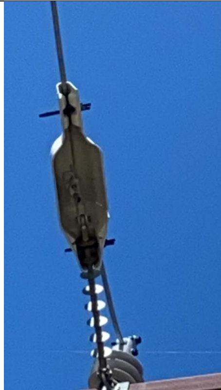
Close up of another dead-end cover having no anti-rotational device
