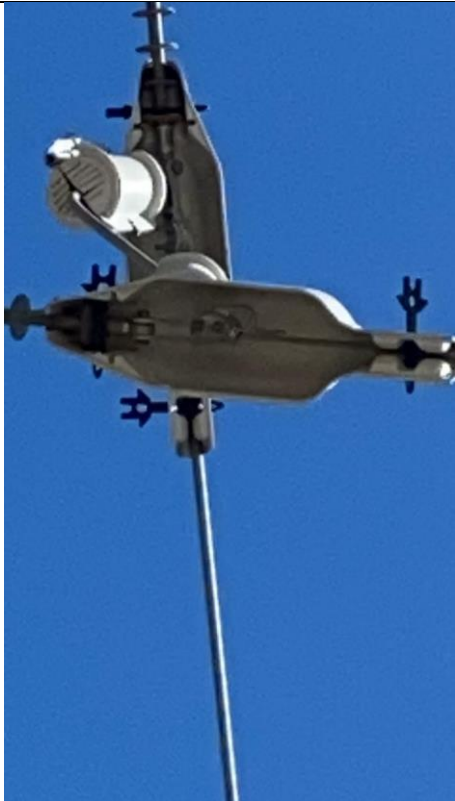
Close up of dead-end cover having no anti-rotational device
