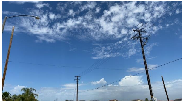
Item6GW1Img2: Overall view of guy span connecting to support pole
