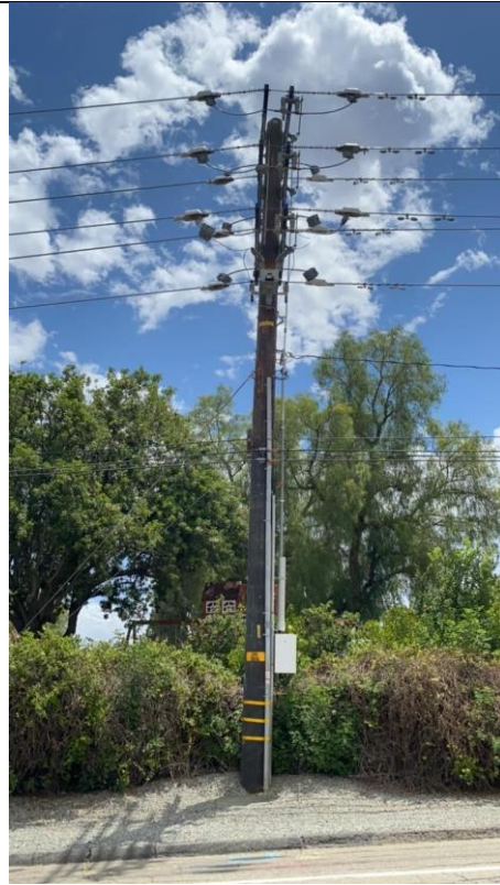
Item8GImg2: Overall pole
