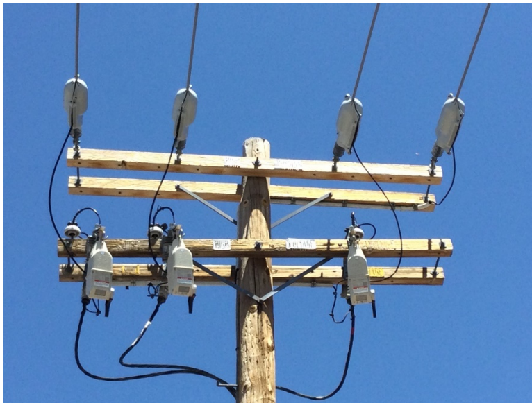
Figure 3-6 — Representative Photo of a TripSaver Fuse Installation
