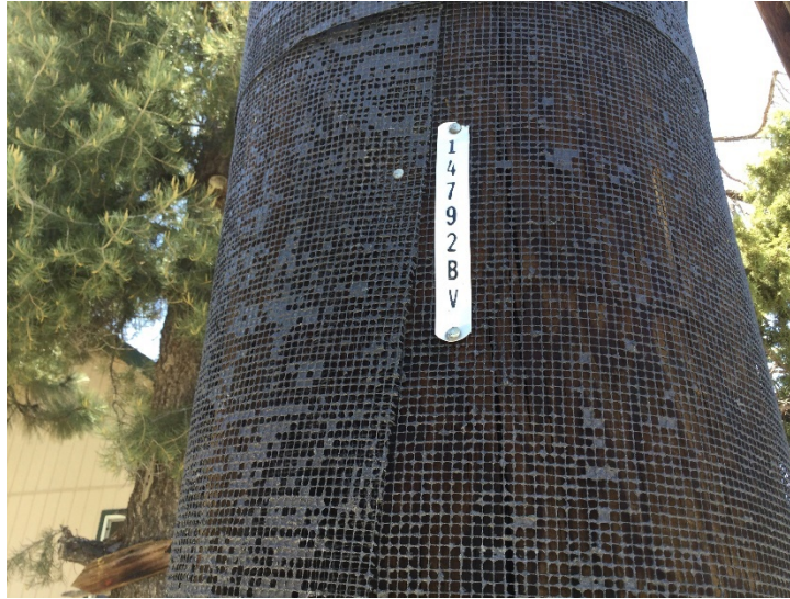
Figure 3-8 — Representative Photo of a Pole Fire Wrap Installation
