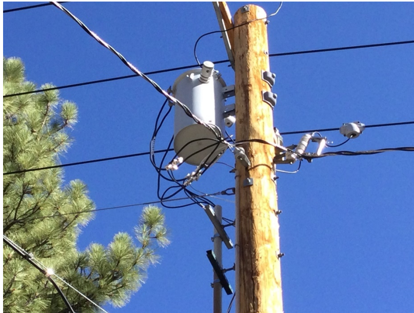
Figure 3-4 — Representative Photo of an ELF Fuse Installation
