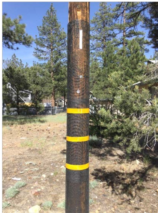
Figure 3-8 — Representative Photo of a Pole Fire Wrap Installation
