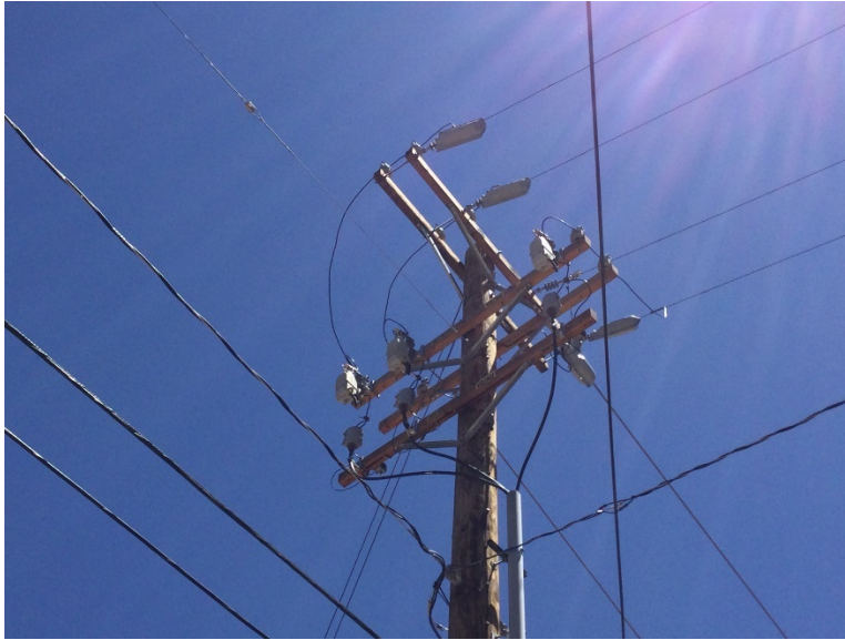
Figure 3-6 — Representative Photo of a TripSaver Fuse Installation
