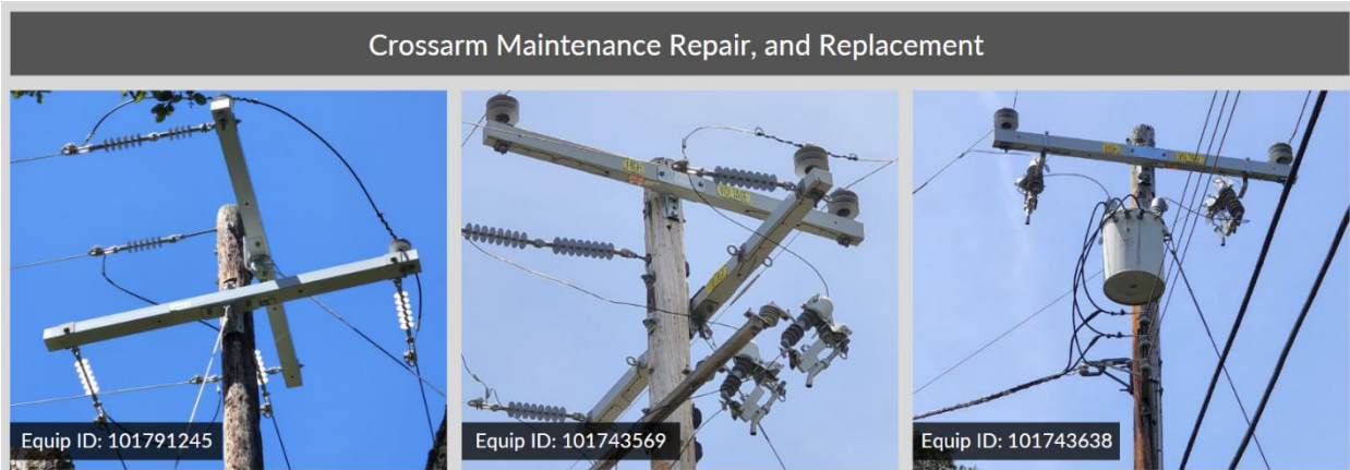
Figure 13: Example Crossarm Maintenance Repair and Replacement Field Images
