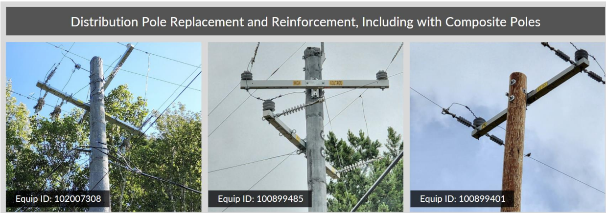
Figure 14: Example Distribution Pole Replacement and Reinforcement, Including Composite Poles Field Images
