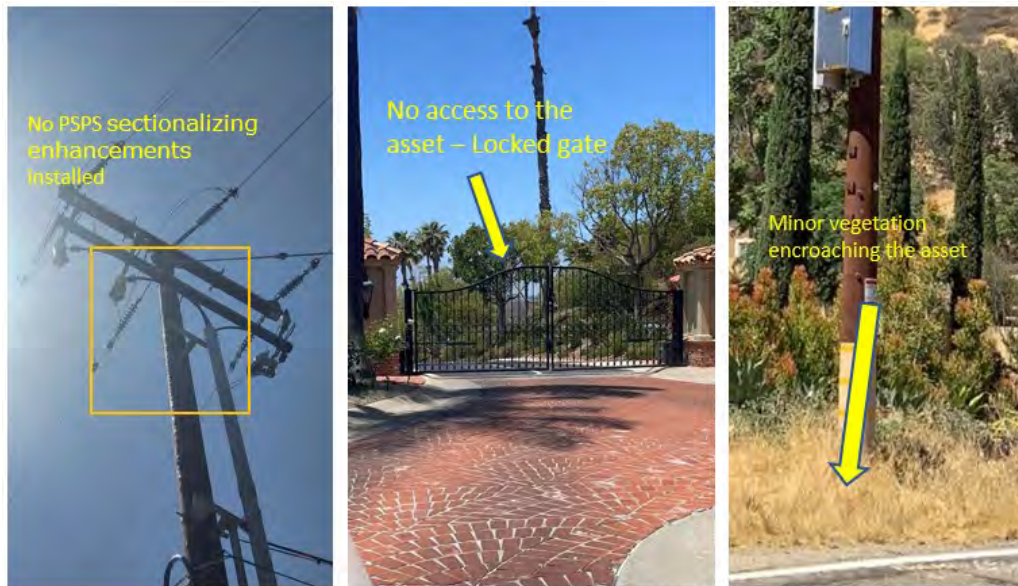
Image 45: Sectionalizing Enhancements with issues.
