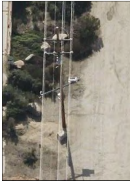
7.1.5. ELM weather station – south
