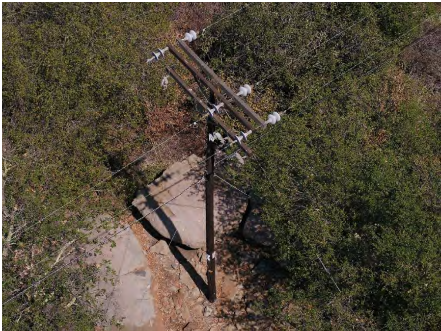
Image 38. Drone image of pole P115803
