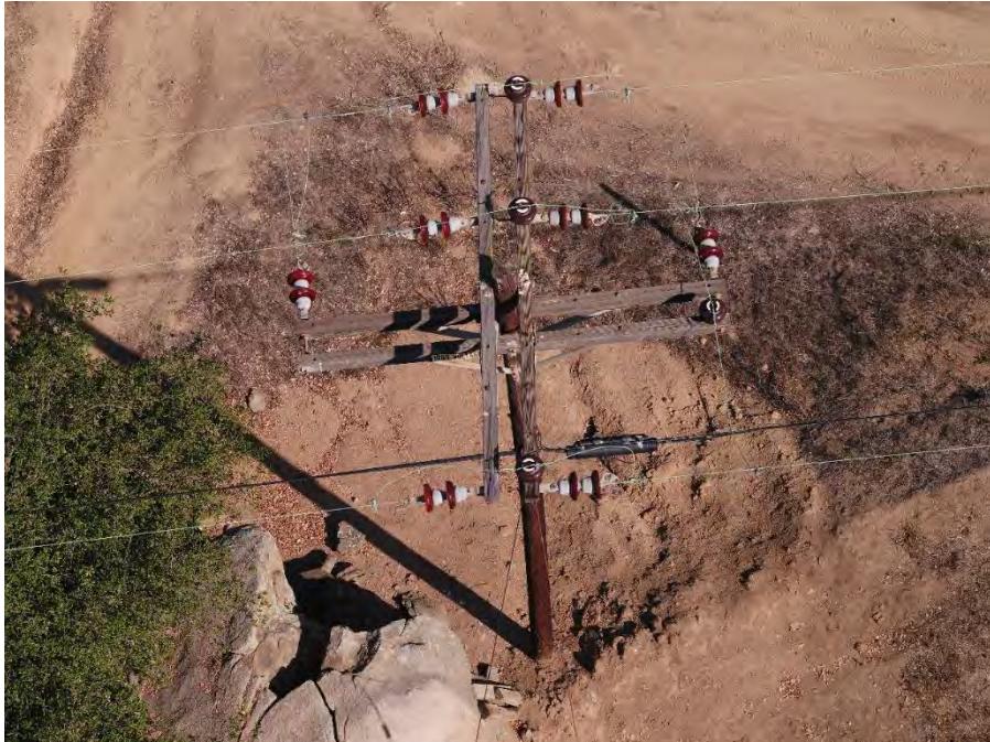
Image 37. Drone image of pole P115804
