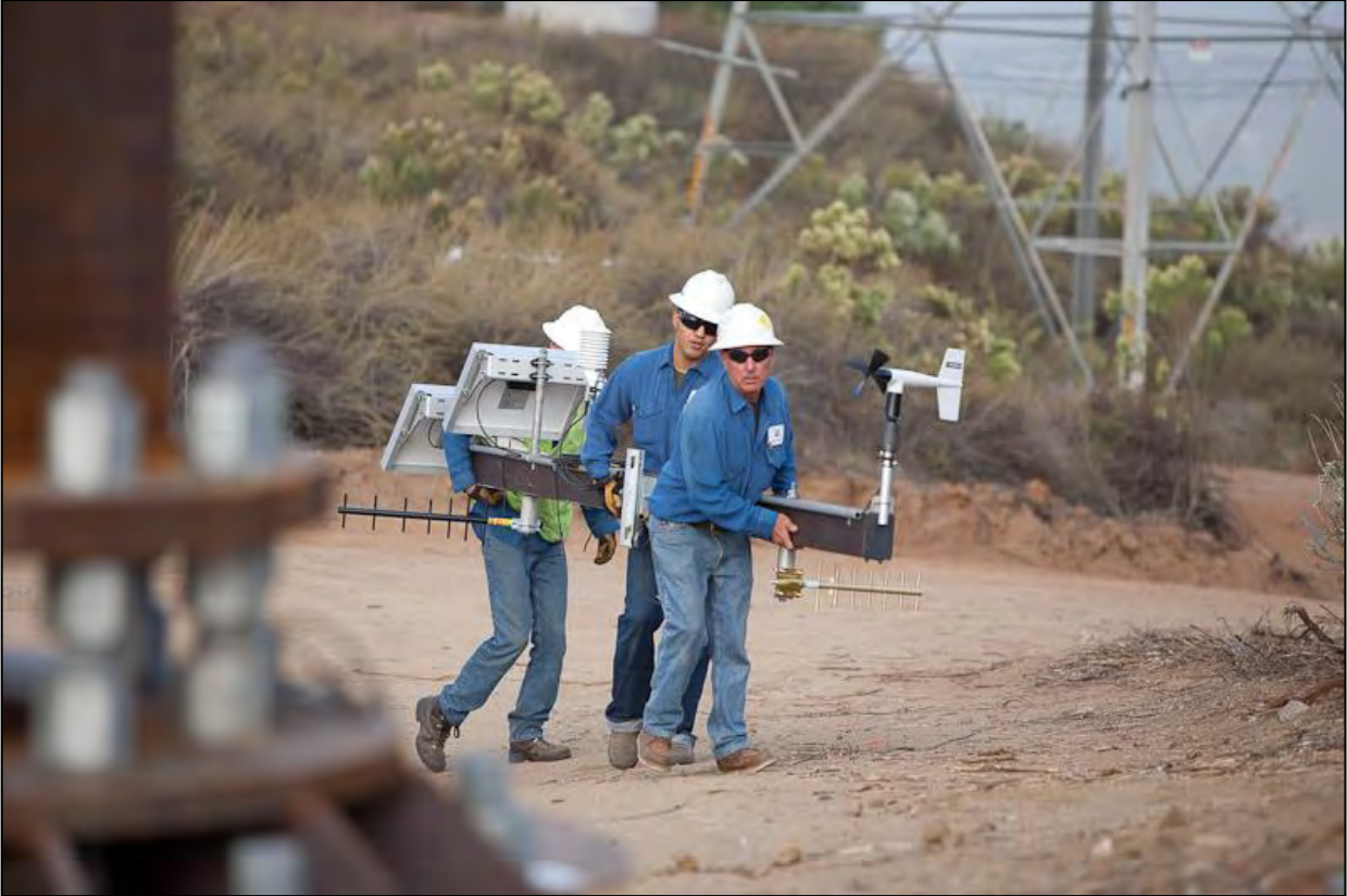
Image 9. Installation of weather station ( source: https://www.sdgenews.com/article/sdges-weather-station-network-has-expanded )
