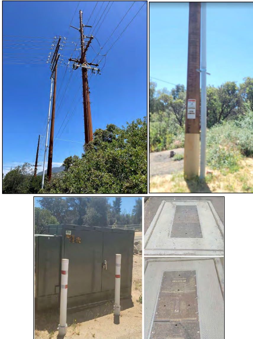
Image 12: No significant findings on transition pole P294891.
