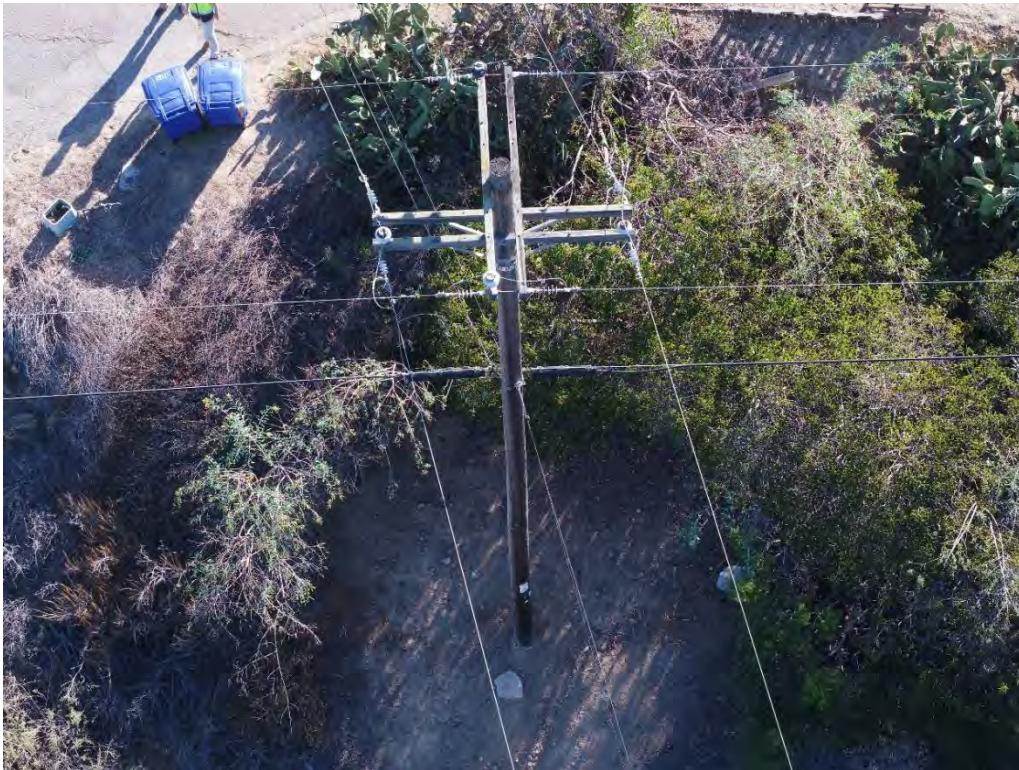
Image 36. Drone image of pole P711567
