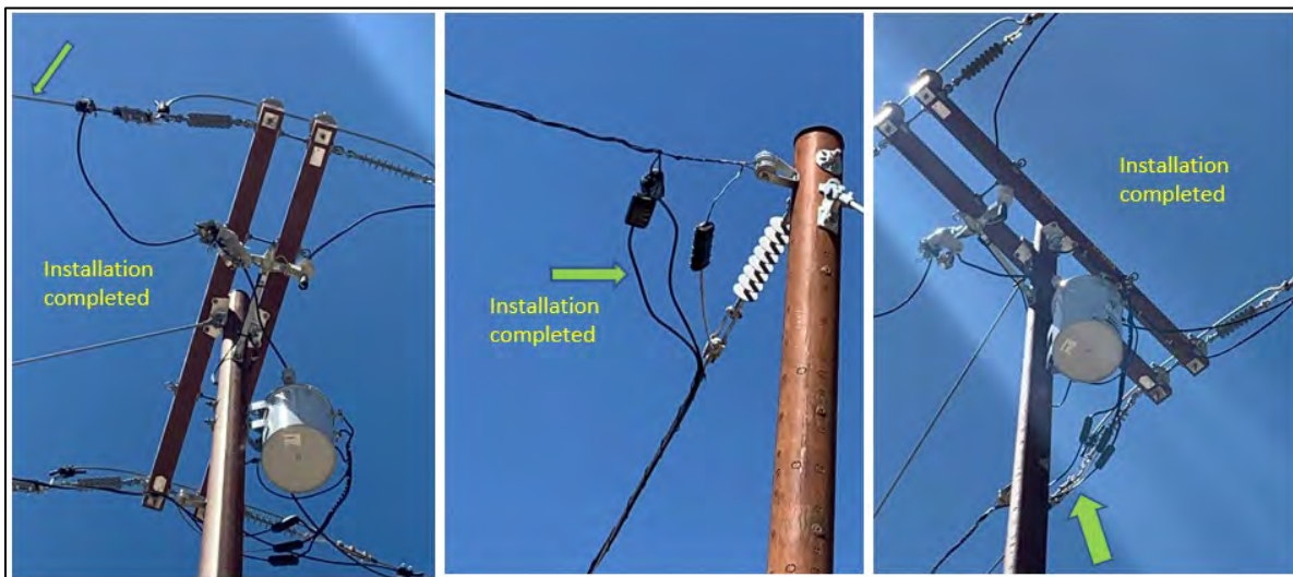
Image 5: Covered conductors installed
