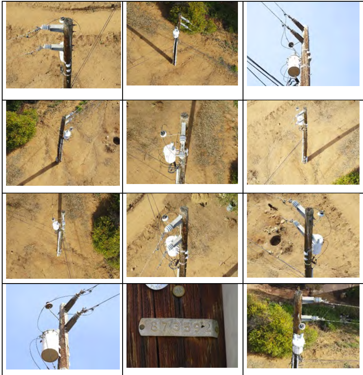
Image 35: Aerial Pole Imagery.
