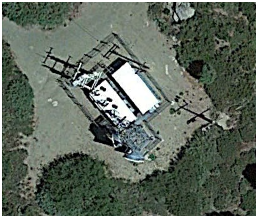
Image 9. Base station with multiple antenna
