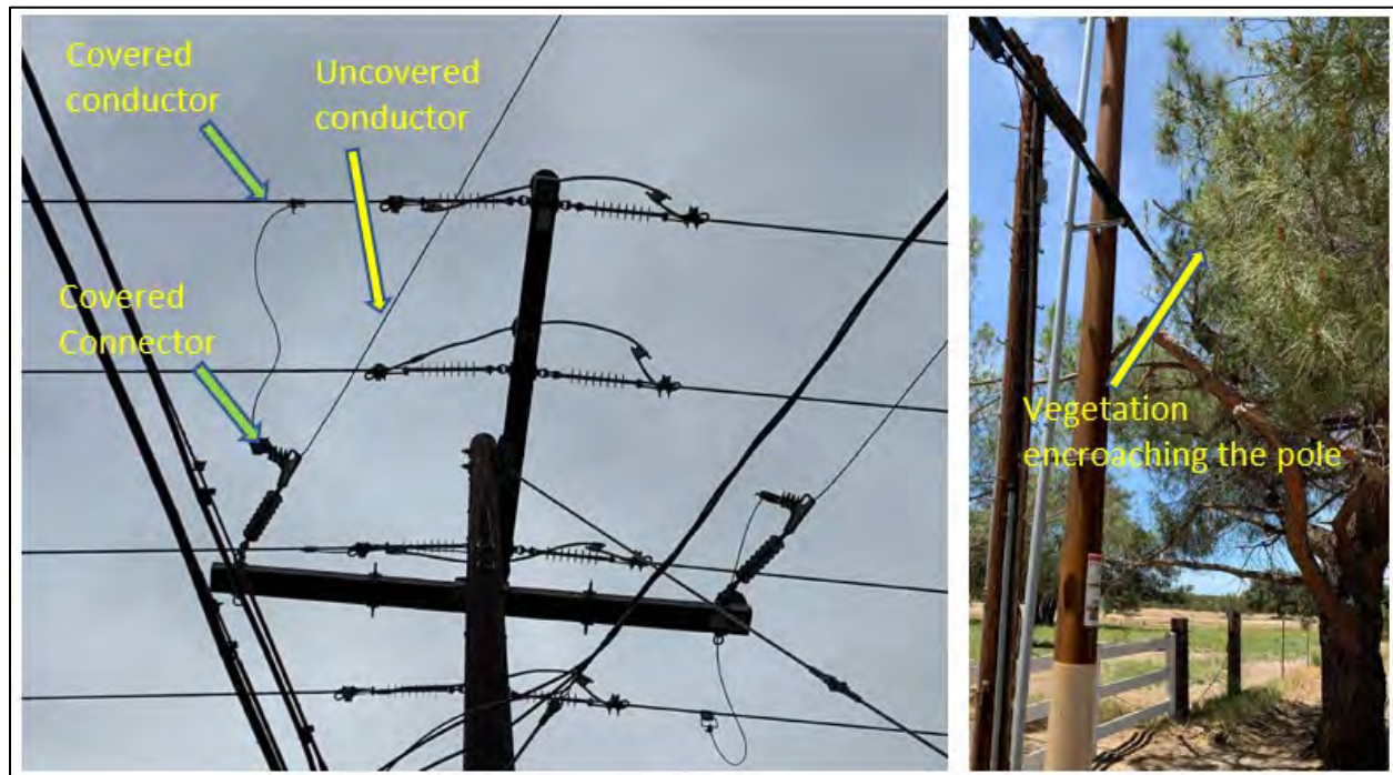
Image 15: Overhead hardening verification with observations.
