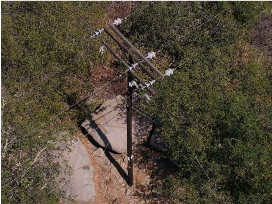
Image 38. Drone image of pole P115803
