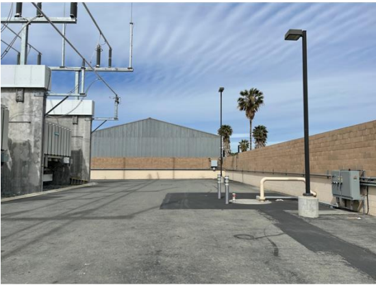
Appendix Figure 5. 230/180-kV transformers
