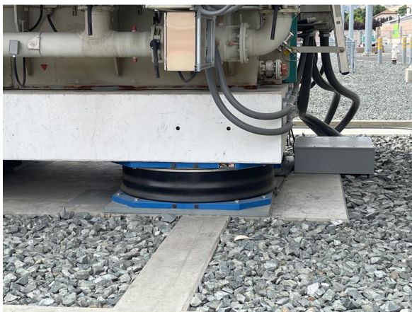
Figure 112: Seismic Base Isolator
