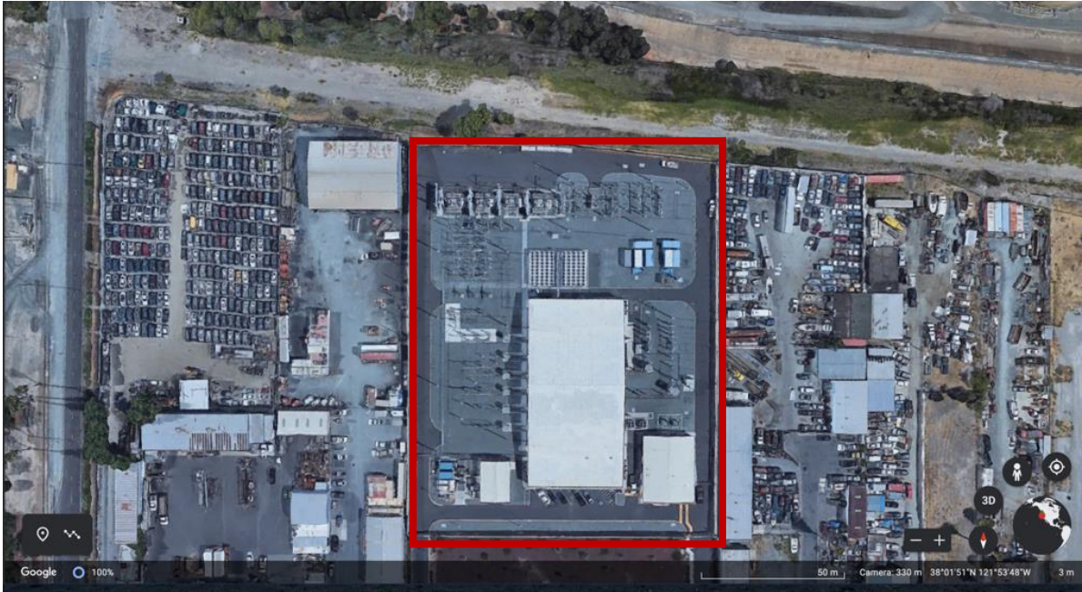
Figure 5: Overview of TBC Pittsburg Facility
