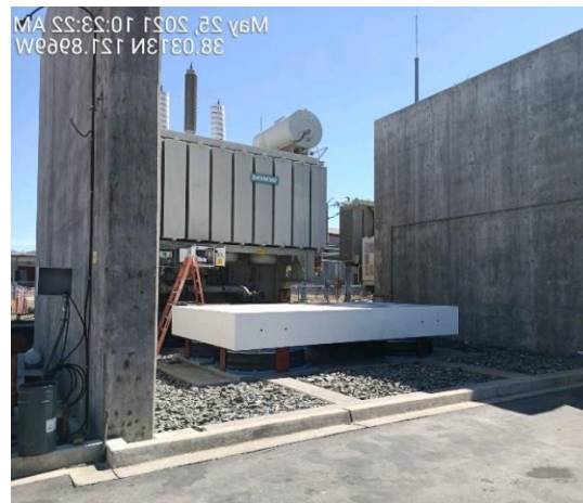
Figure 13: Seismic Upgrade Construction
