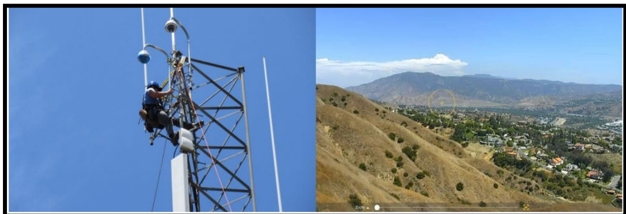
Figure 5 (b) High Resolution Camera Installation and Camera Image Overlooking Anaheim.
