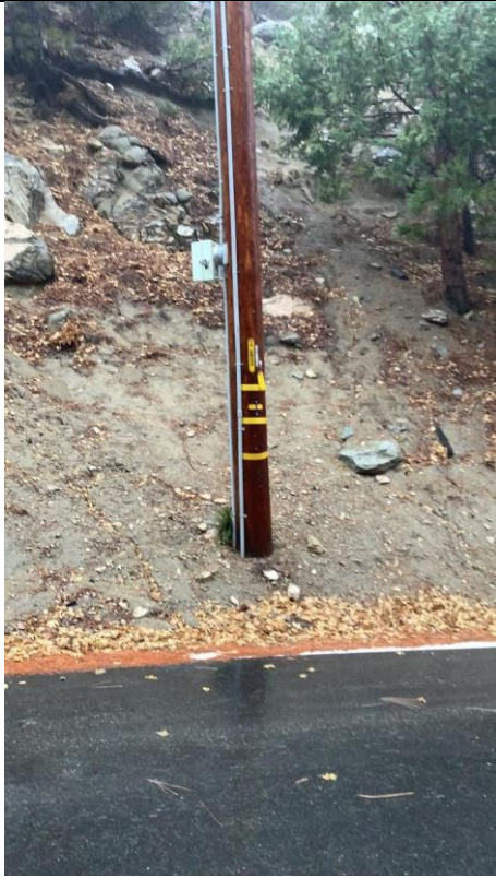
Item3GImg3: Base of Pole
