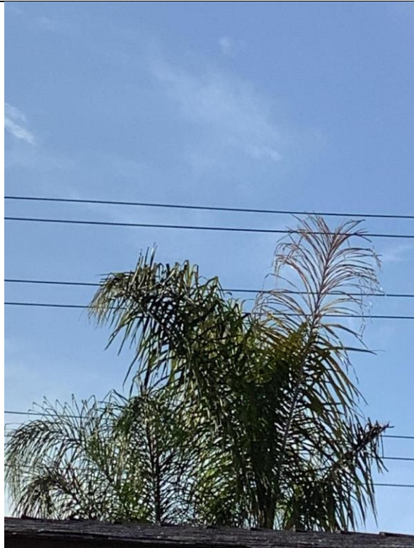
Item9IA1Img3: Palm fronds contacting conductor
