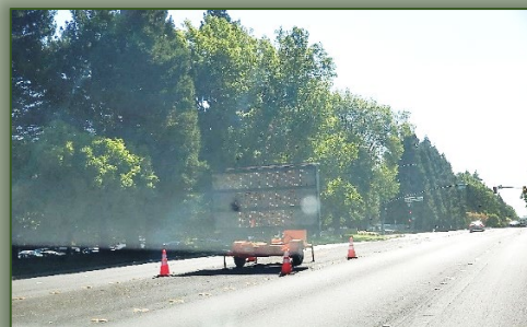
Shown: PG&E Signs Directing Traffic
