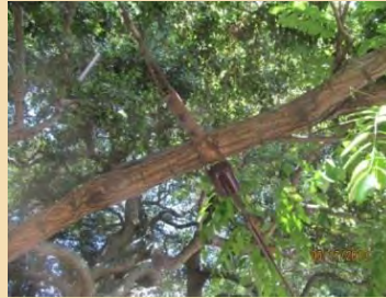
Guy grounded by vegetation
