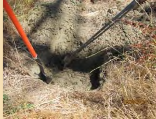
After: Vegetation cleared from anchor
