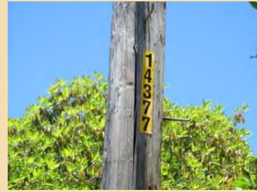
After: Minor work completed, operating number applied below operating position.
