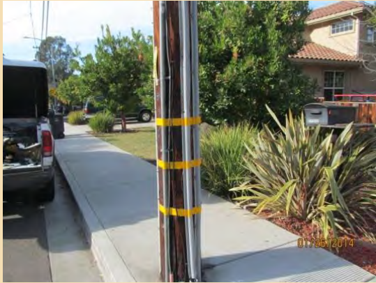
At this Location: Acceptable application of plastic and adhesive visibility strips
