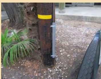
At this Location: Condition acceptable after repair of exposed ground
