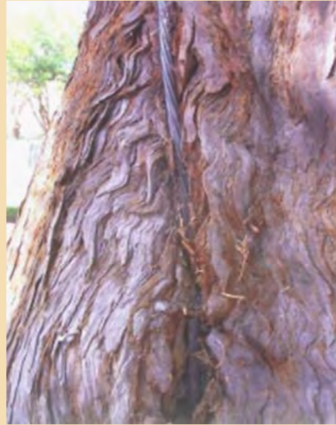
Anchor buried by tree
